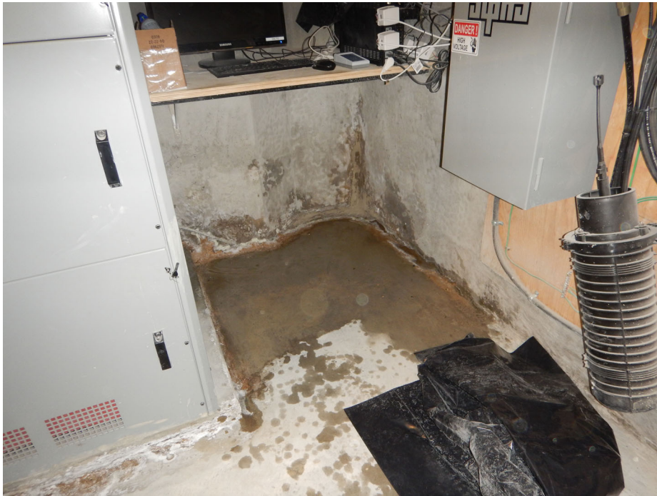
Photo 5: Efflorescence on wall base and water on floor adjacent to equipment (right side).
