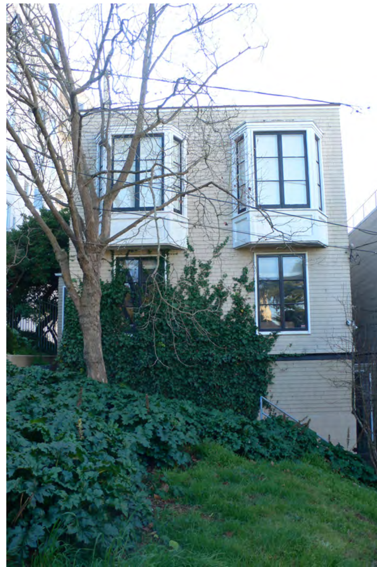
3 FACADE OF SUBJECT PROPERTY SCALE: 1:1.17
