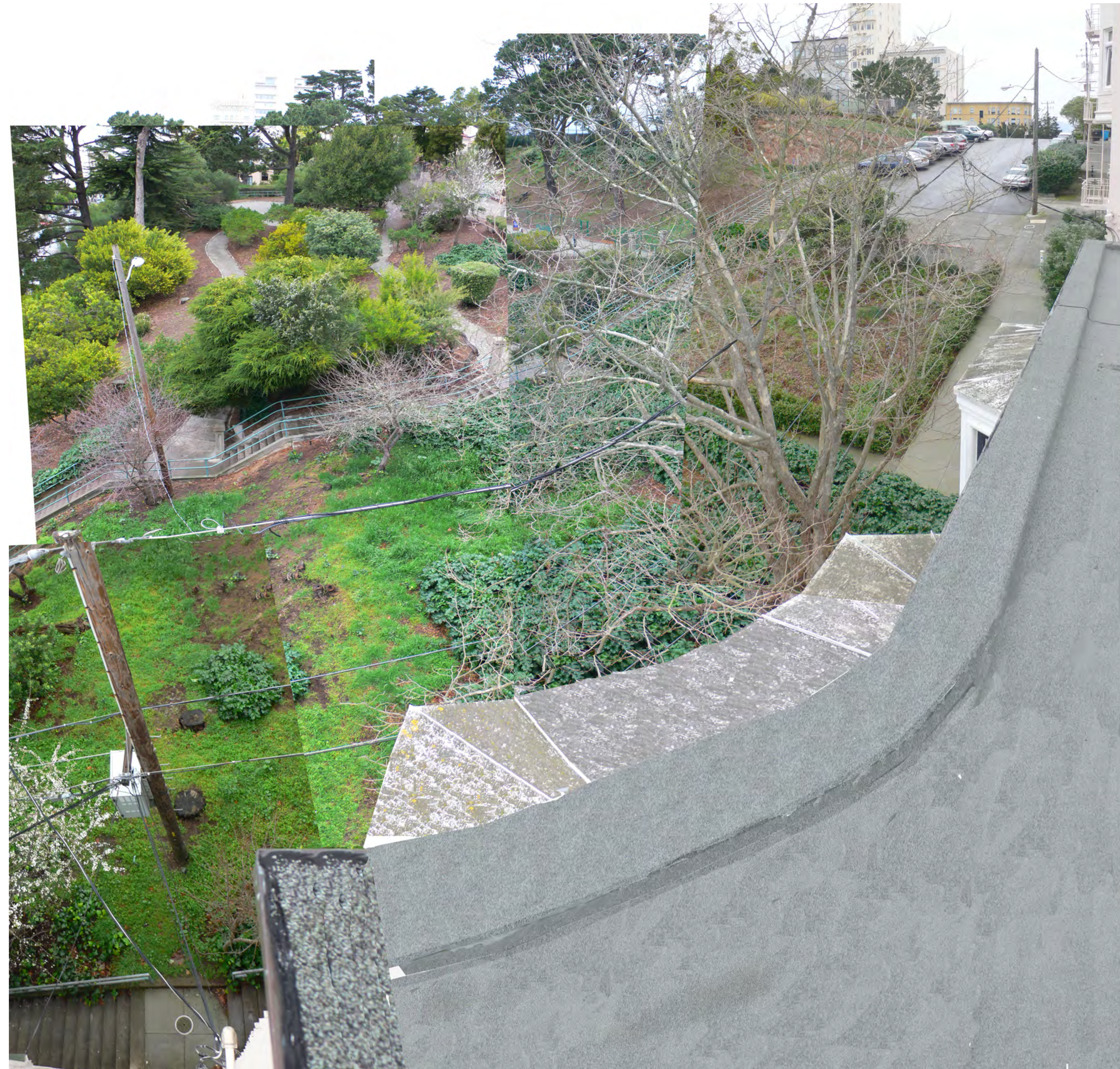
1 EXISTING PARK FROM ROOF OF SUBJECT PROPERTY SCALE: 1:0.54
