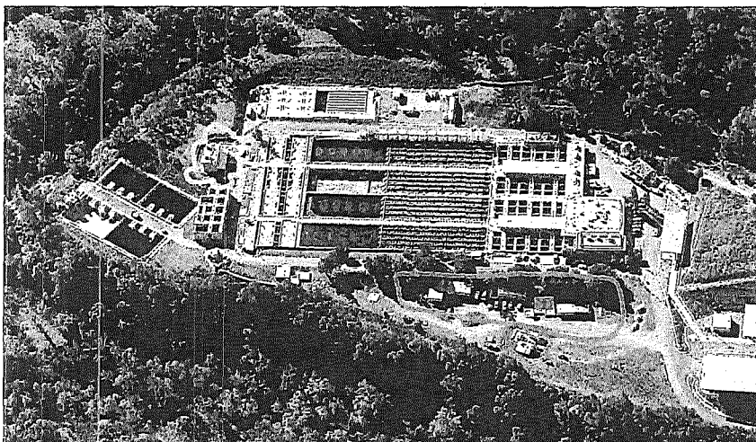
Sunol Valley Water Treatment Plant
