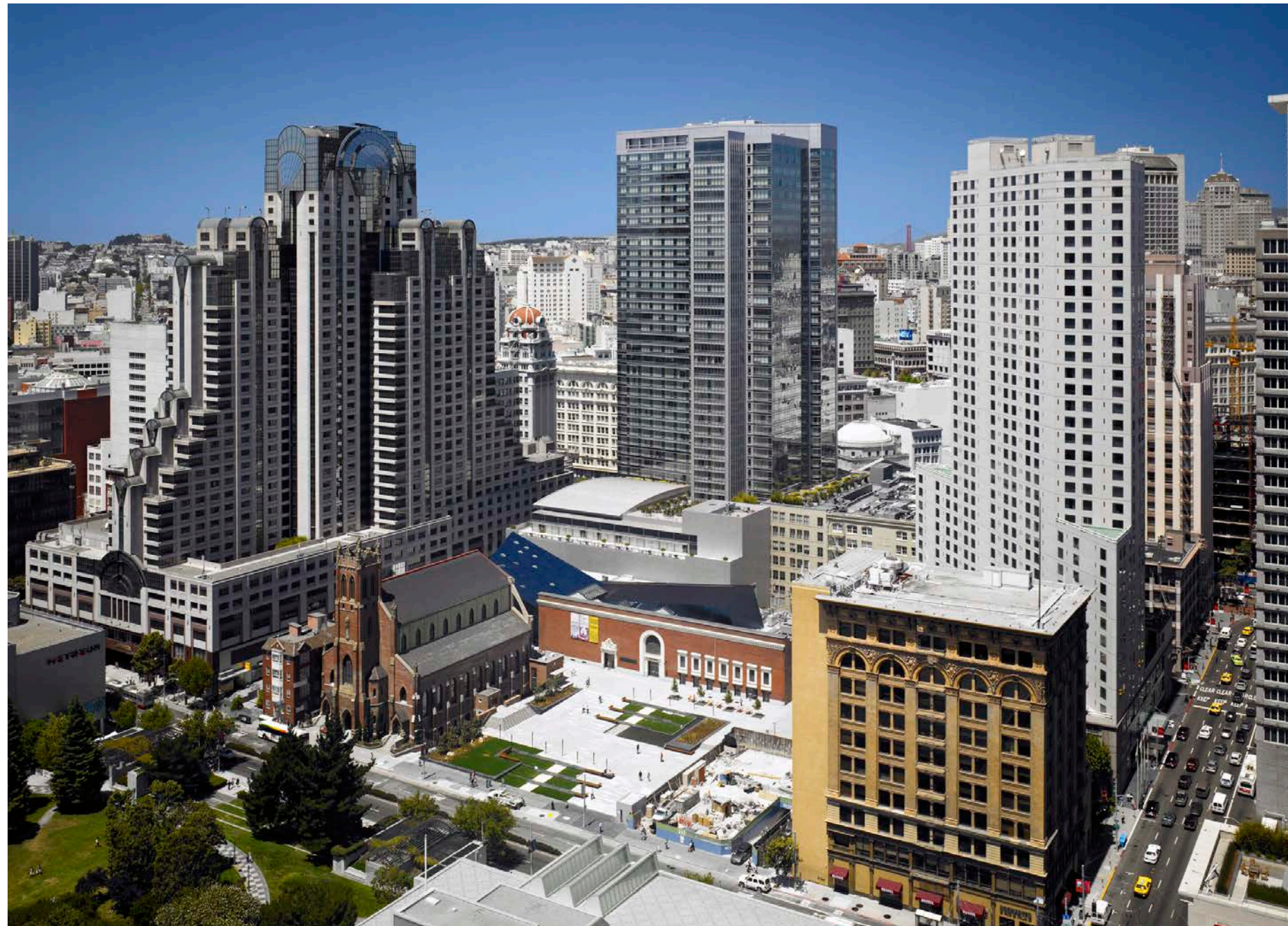
View, looking northwest, 2012. (Handel Architects)
