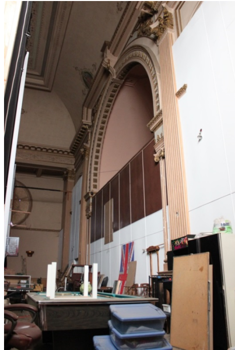
FIGURE 32. CHURCH: SANCTUARY SHOWING SEALED ALTAR NICHES, 2016.
