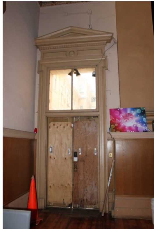
FIGURE 31: CHURCH: NAVE, SOUTH TRANSEPT ENTRY TO ALLEY, 2016.
