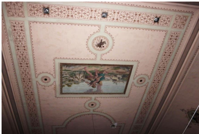
FIGURE 29. CHURCH: NAVE, WEST PORTION OF PAINTED CEILING, 2016.
