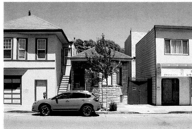
3 SUBJECT PROPERTY FRONT FACADE
