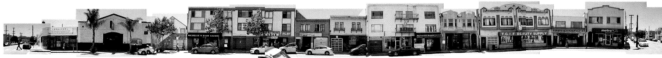
2 SAN BRUNO STREET FACING WEST
