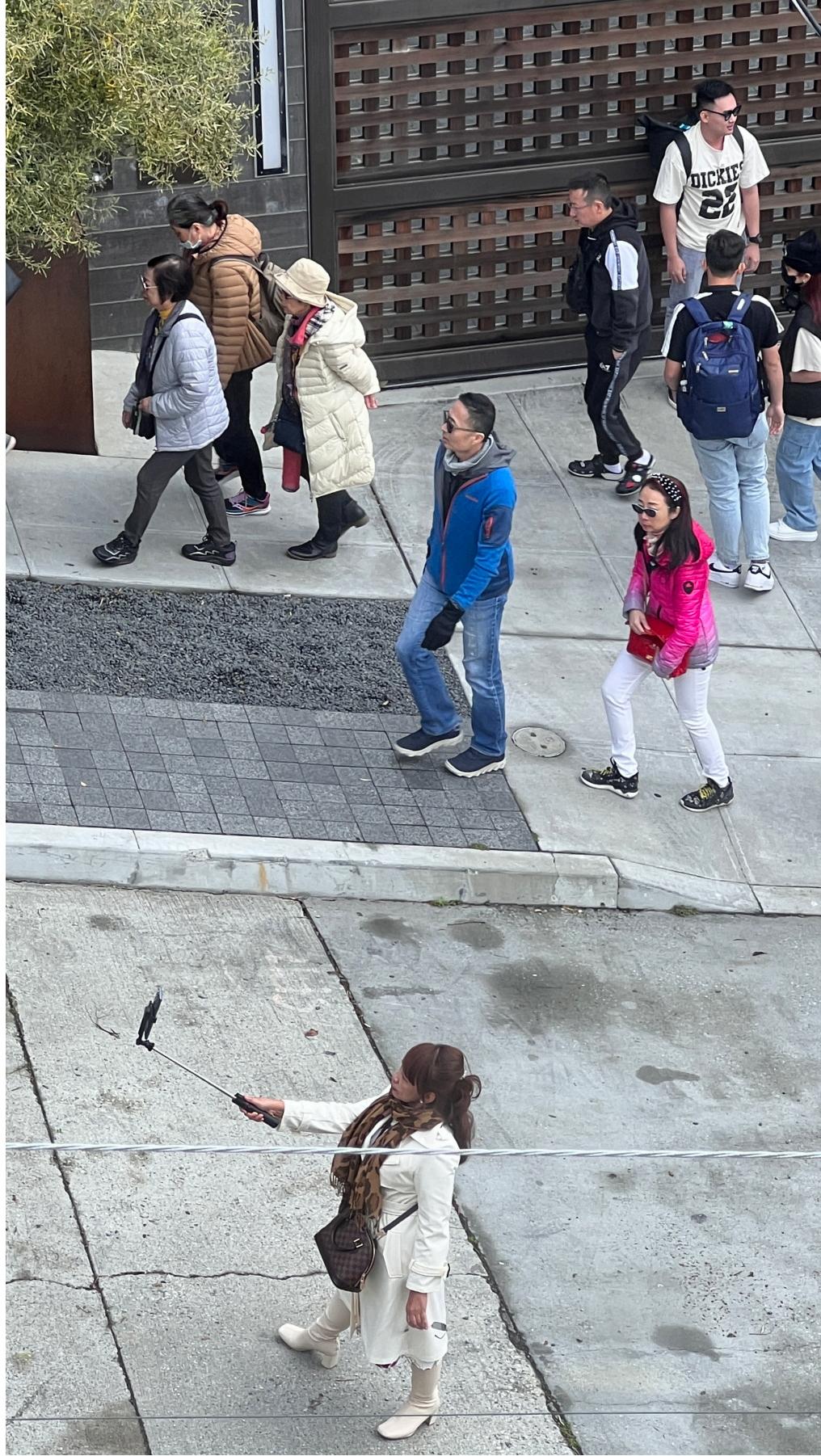
Tourists and locals and school children have to jaywalk. No one wants to walk on the construction side of the new building. Accidents do happen.
