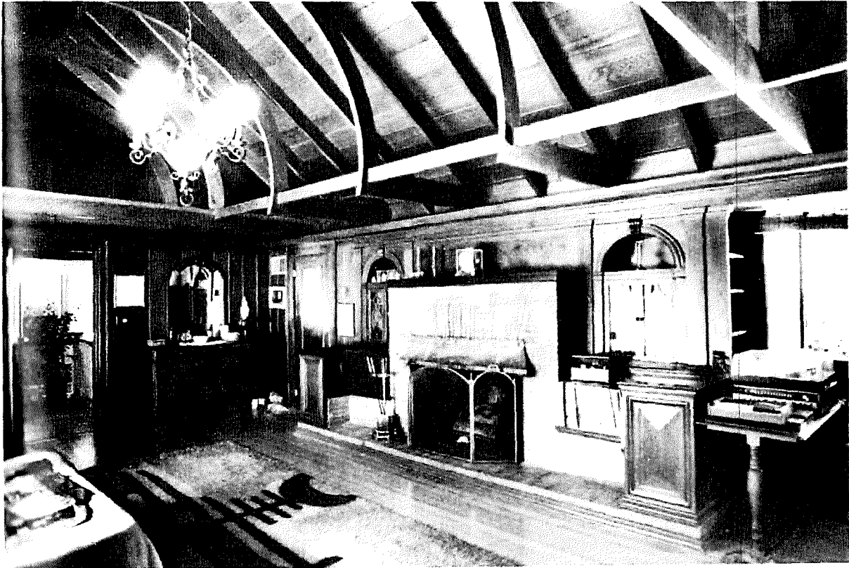
Figure 19. Unique exposed truss details, first experimented with in the studio of the Ernest Coxhead Residence and Studio ( Photo 29 ) becomes a featured detail in a project for Frank Washington built at few years later in Mill Valley, California (Longstreth, p. 171).
