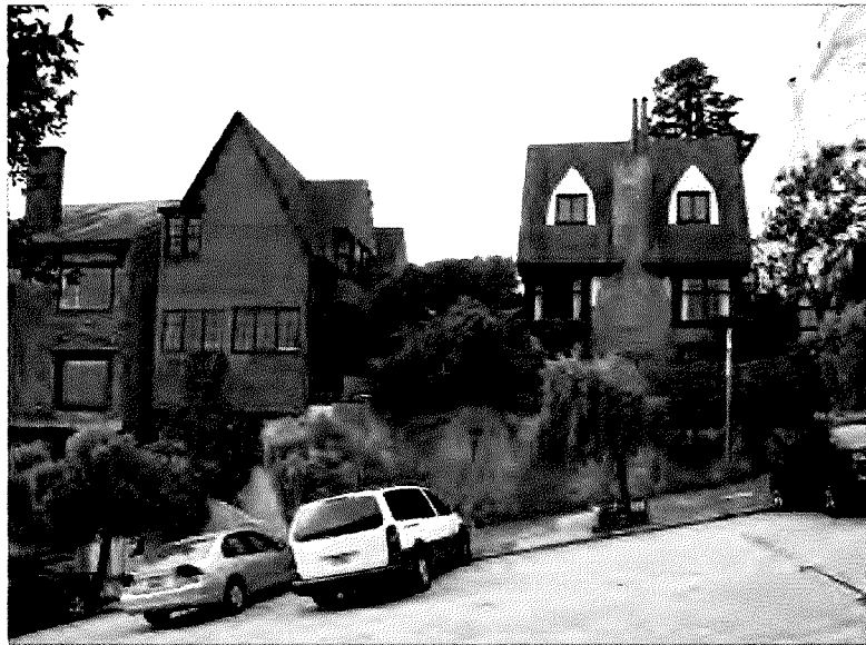
Coxhead's own home at 2421 Green (left) and his design next door at 2423 Green would have been new and somewhat daring within the Victorian landscape of the time.
