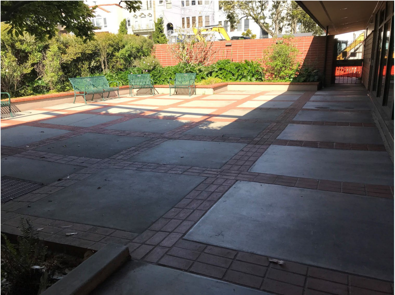
Parkside Branch Library, terrace at north side of building, view northeast, 2023. Source: San Francisco Planning Department
