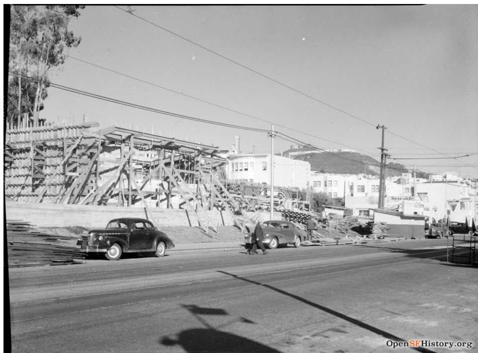
Parkside Branch Library, under construction, 1950. Source: Western Neighborhoods Project, OpenSFHistory / wnp28.0034
