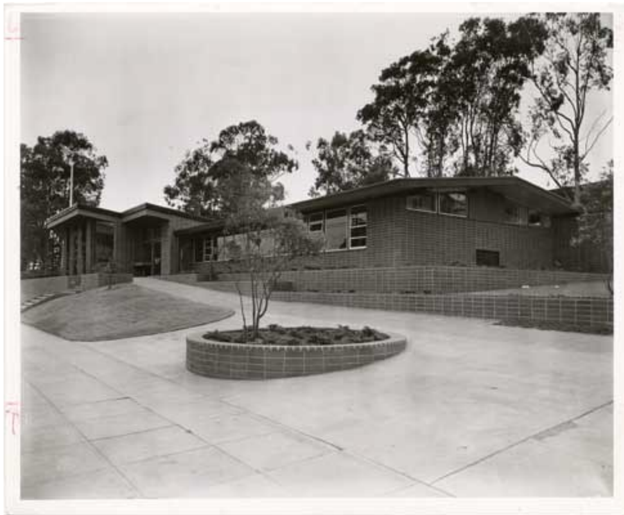
Parkside Branch Library, view northwest, June 19, 1951.
