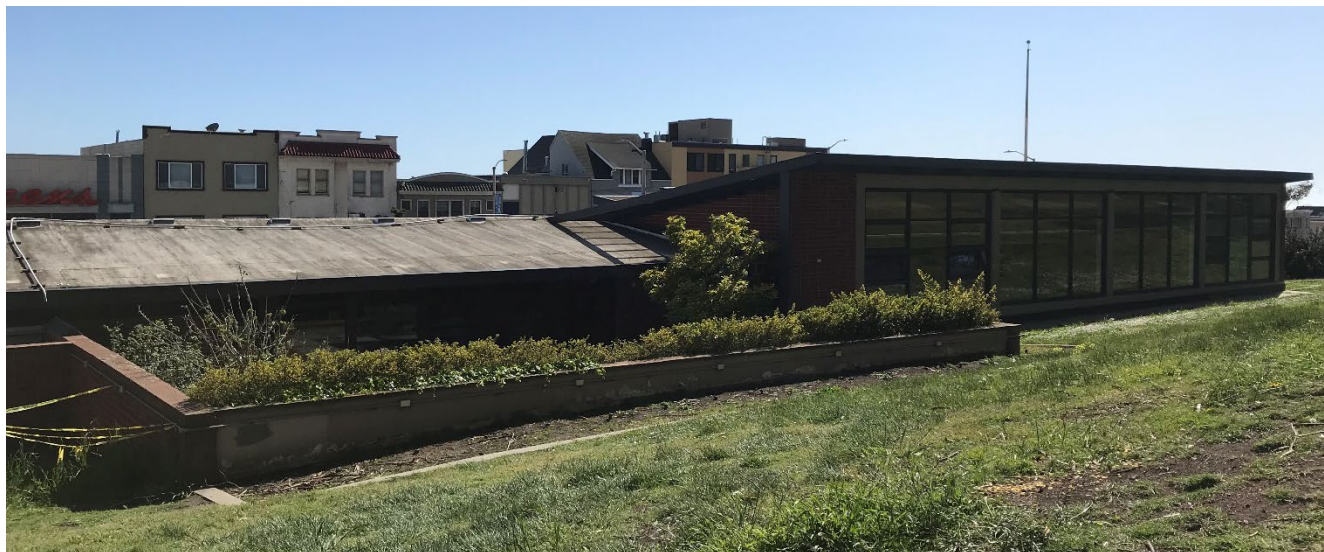
Parkside Branch Library, north elevation, view southwest, 2023. Source: San Francisco Planning Department
