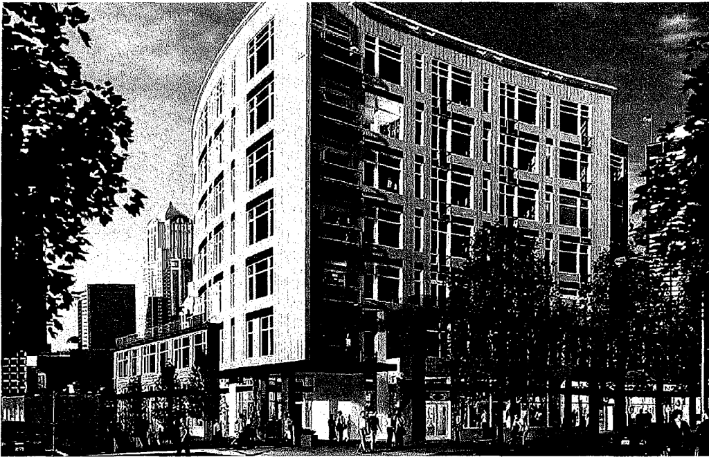
The Landes is an example of a five-story woodframe building over two stories of concrete, a common construction type for Seattle, but not San Francisco.
