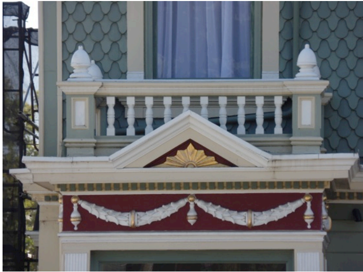
Figure 10. Detail of balustrade over entrance portico. (Photograph by Garavaglia Architecture, Inc., April 2015.)
