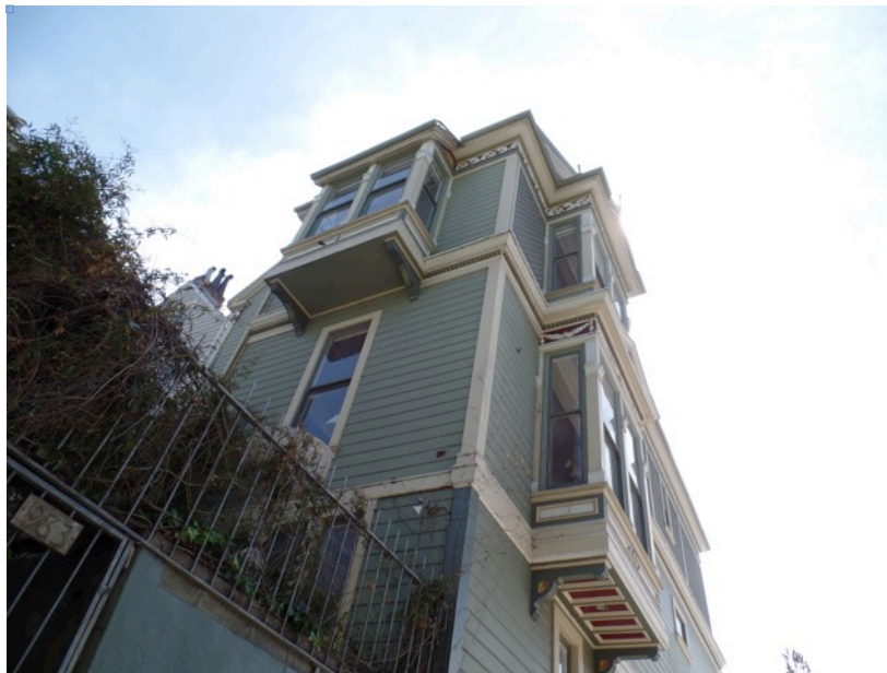
Figure 13. Partial view of the east (rear) elevation. (Photograph by Garavaglia Architecture, Inc., May 2015.)
