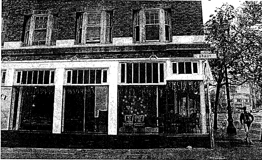
Figure 11 - 1649 Market Street, storefront detail
