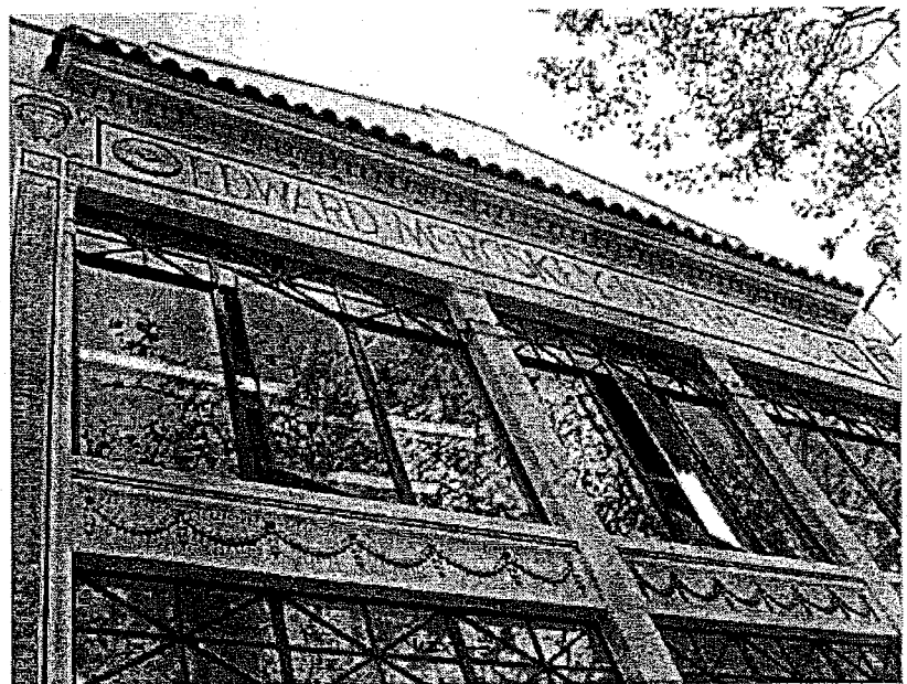
Figure 24 - 1687 Market, upper floor detail
