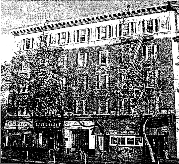
Figure 8 - 1649 Market Street, Market Street elevation
