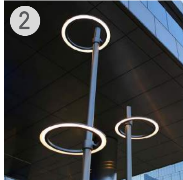
2 Landscape Forms: “Typology Ring” Overhead light fixtures.
