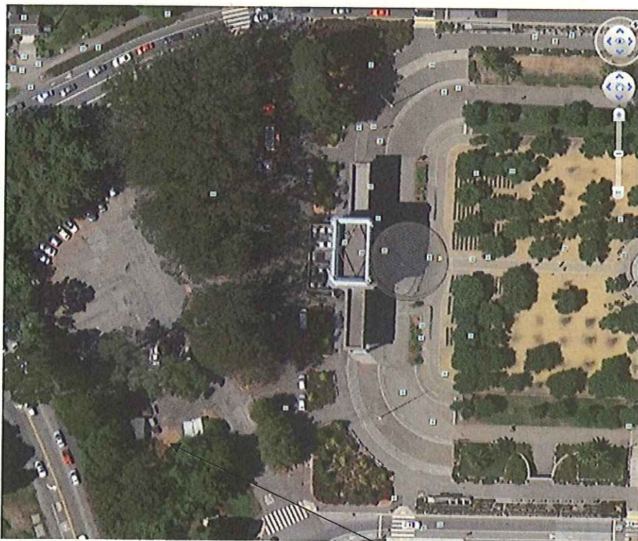
Four additional storage containers to be added.
