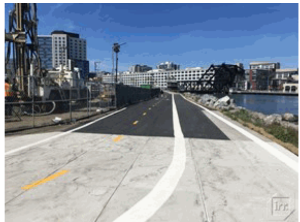
Facing West Along McCovey Cove
