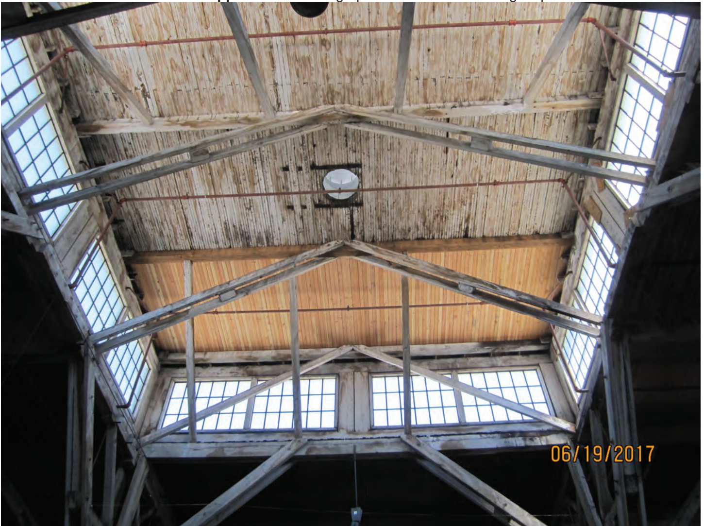
Photo 10. Roof monitor with new beam and 2x4 sheathing.
