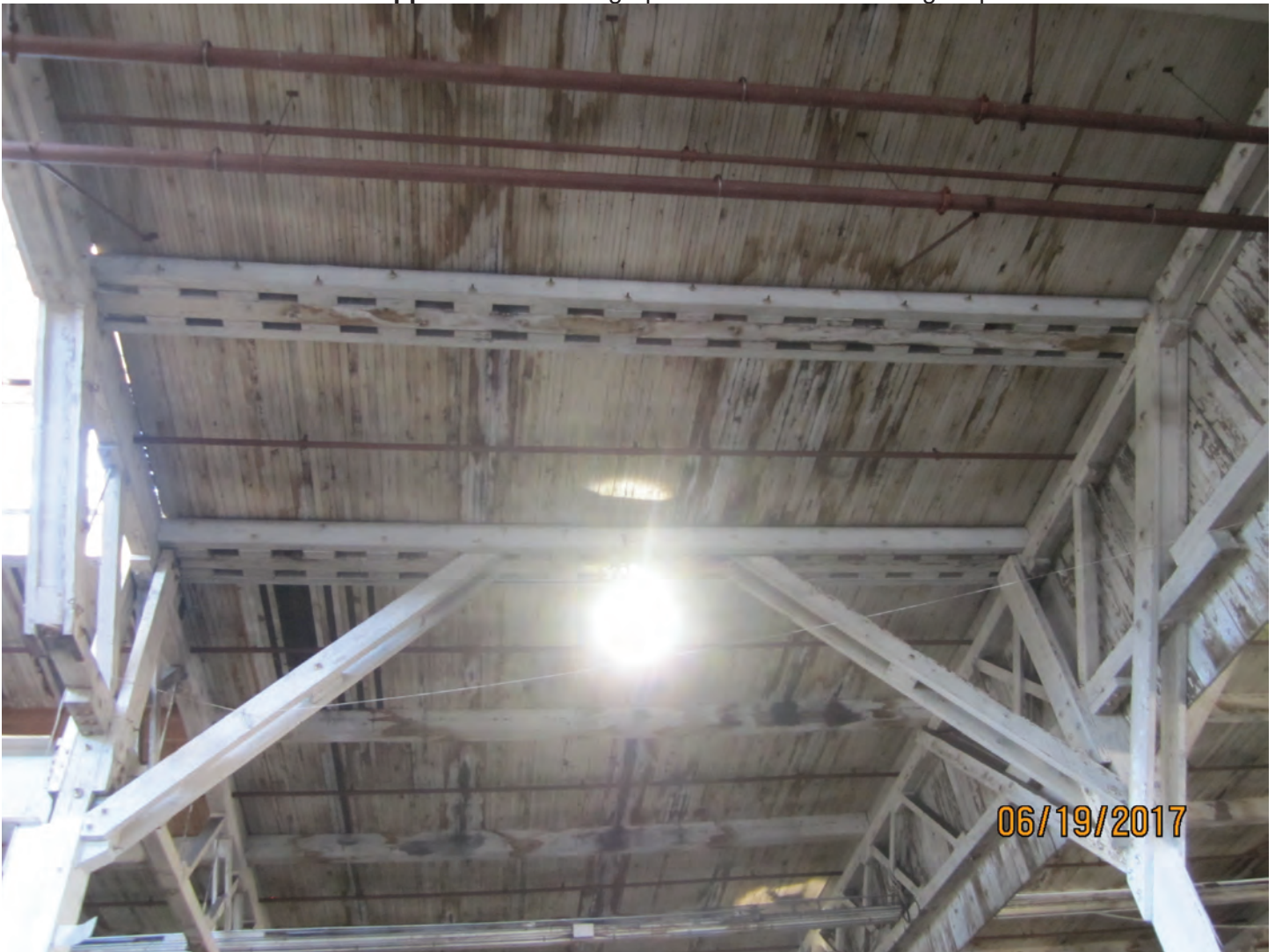
Photo 14. Wood roof beams strengthened in the past.
