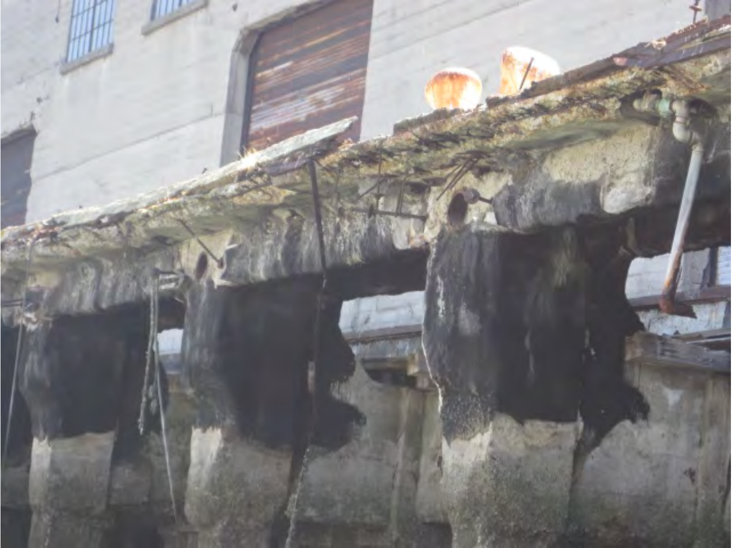
Photo 9. Deteriorated deck
