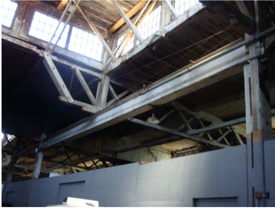
Photo 5. Repair work with steel beams after the post removal
