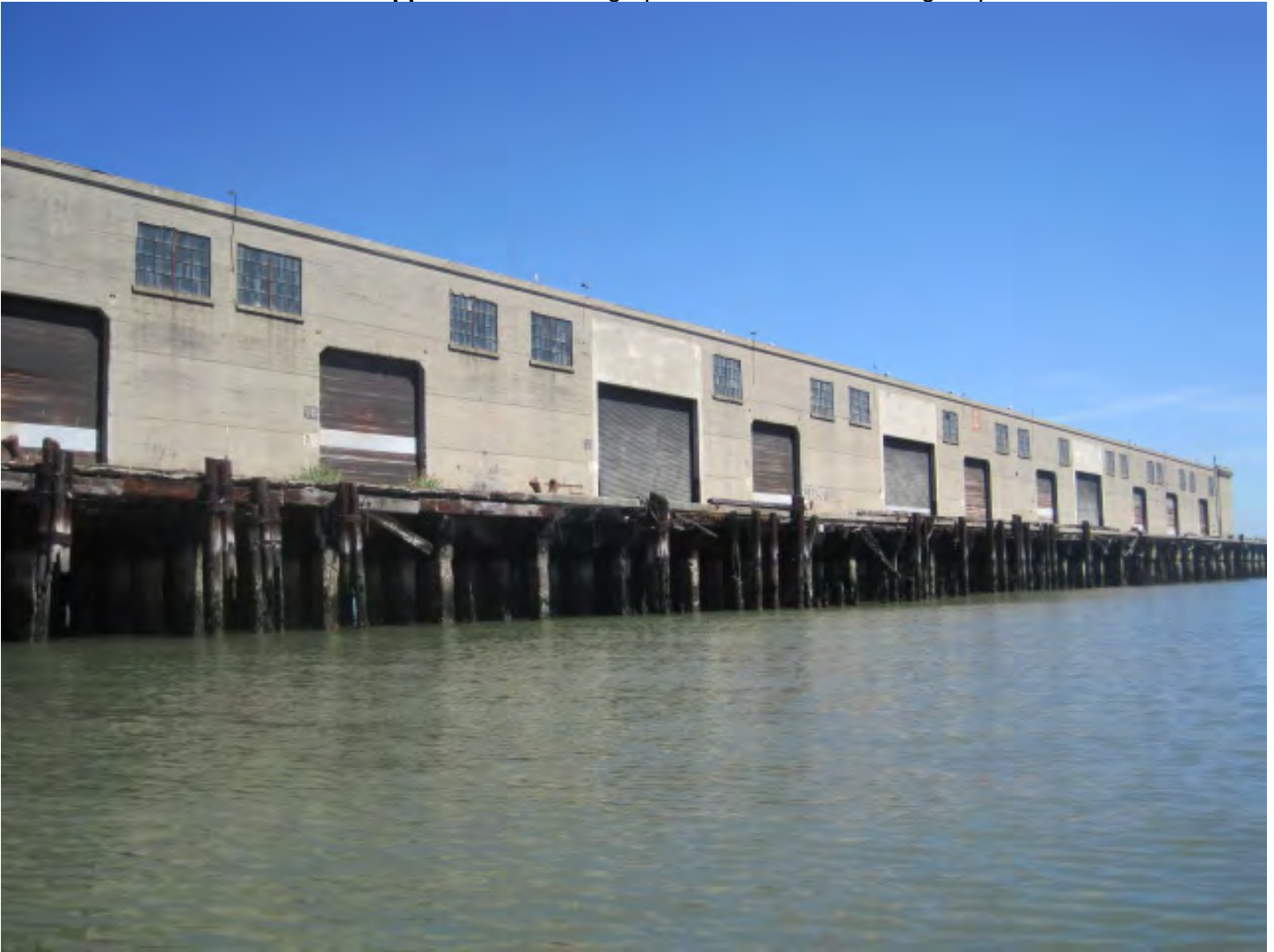
Photo 8. Overall view looking at south side
