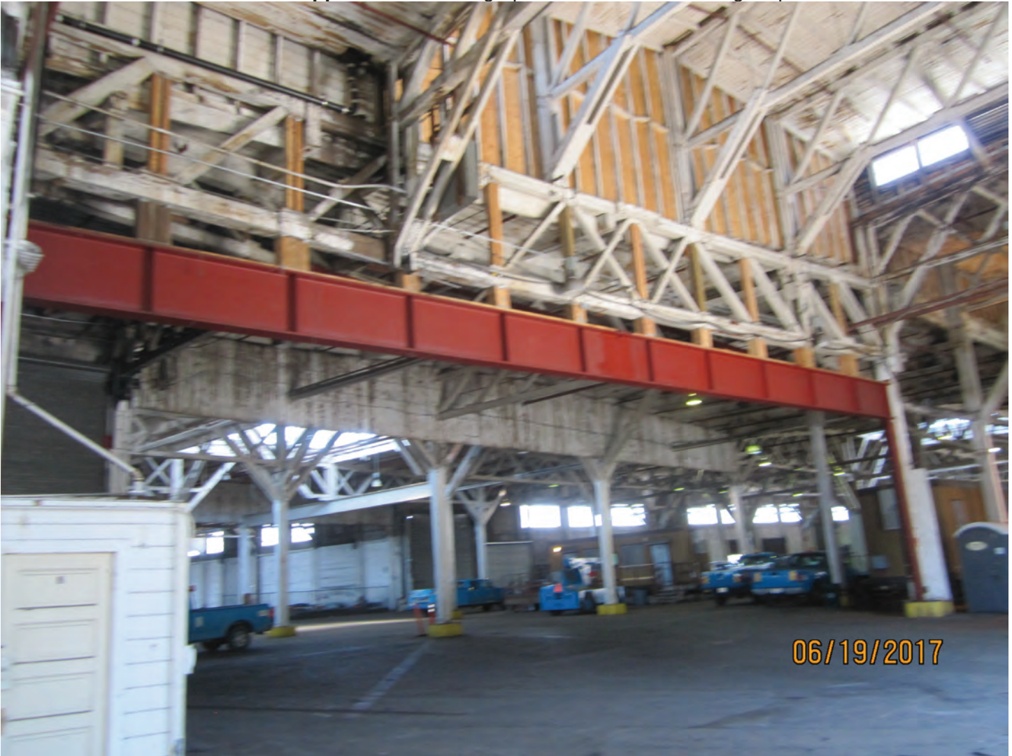
Photo 7. New steel beam and tube steel posts added in 2017 to strengthen existing wood truss.
