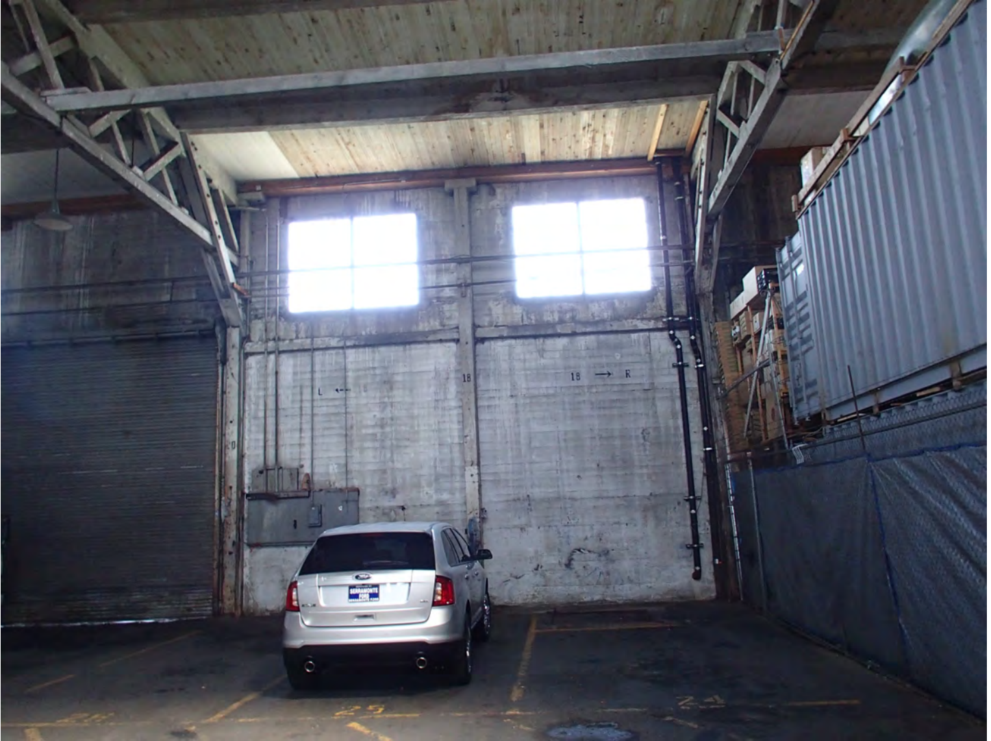
Photo 7. View of the concrete wall with interior wood framing
