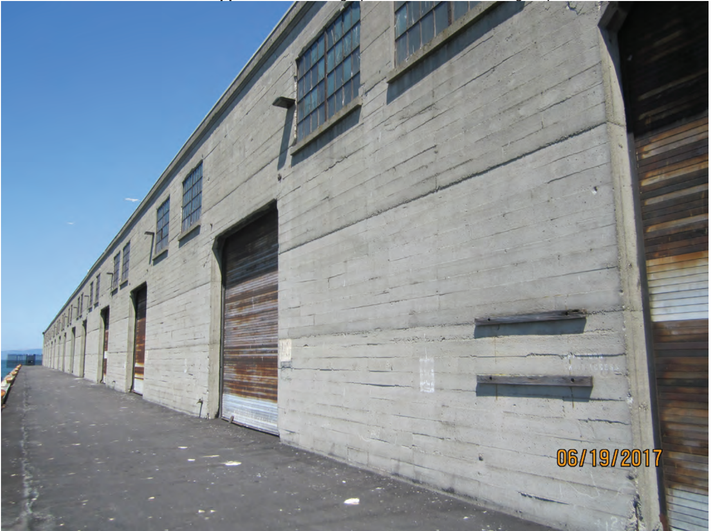
Photo 3. Exterior concrete wall along north face of building.
