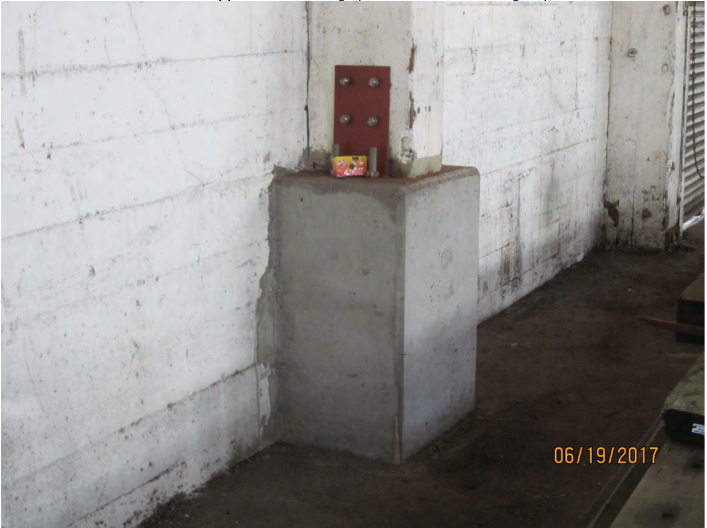
Photo 9. New concrete footings installed to replace dry rotted column bases in 2017.
