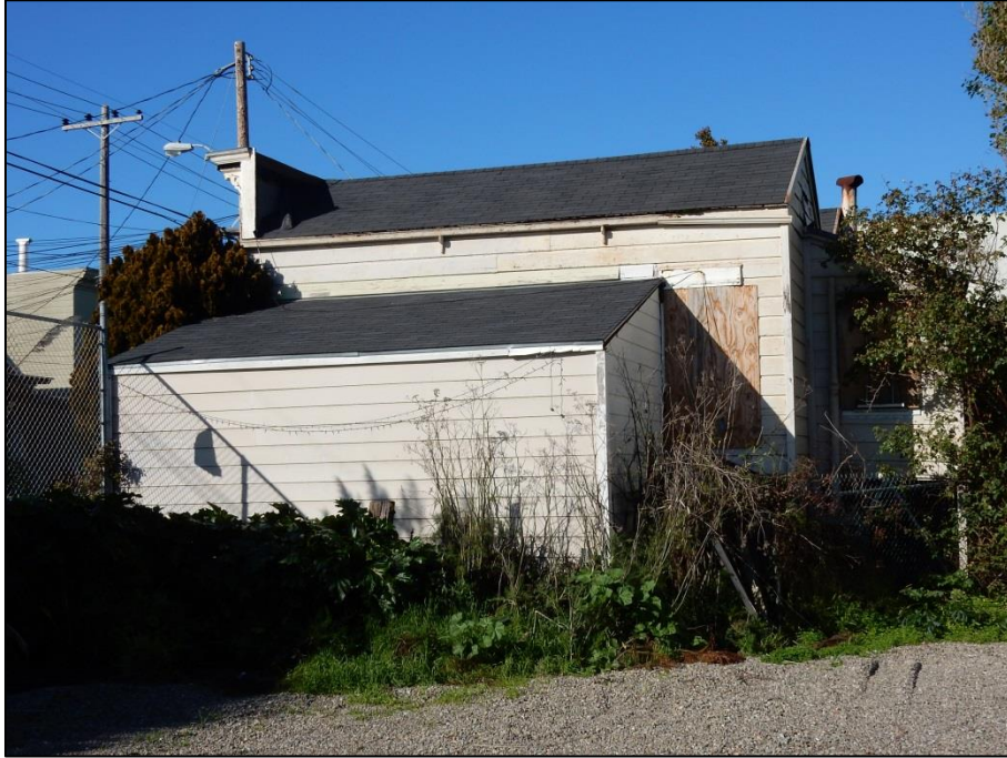
Figure 3 – 953 Treat Avenue – South elevation showing additions to the south.
