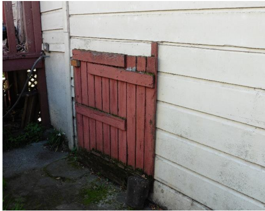
Figure 13. Crawlspace entrance at north façade.
