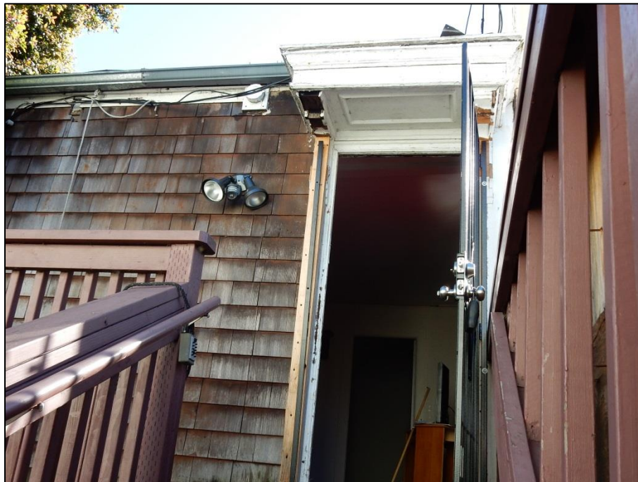
Figure 2 – 953 Treat Ave – North elevation.
