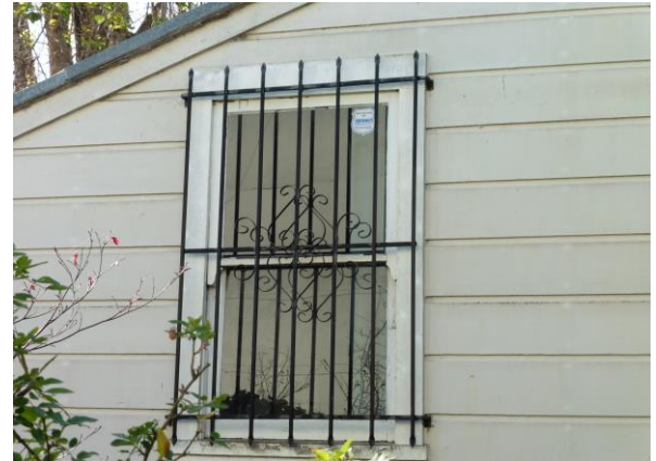
Figure 14. Double hung window in east portion of façade.
