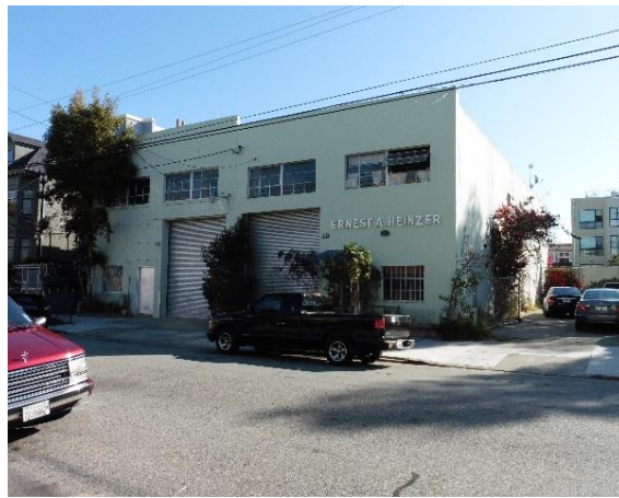
Figure 28. Warehouse north of subject property.
