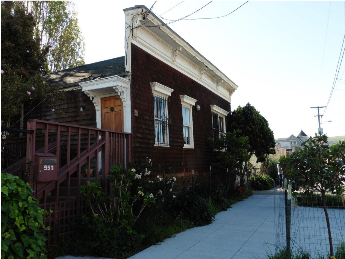
Figure 3. 953 Treat Ave, looking east.
