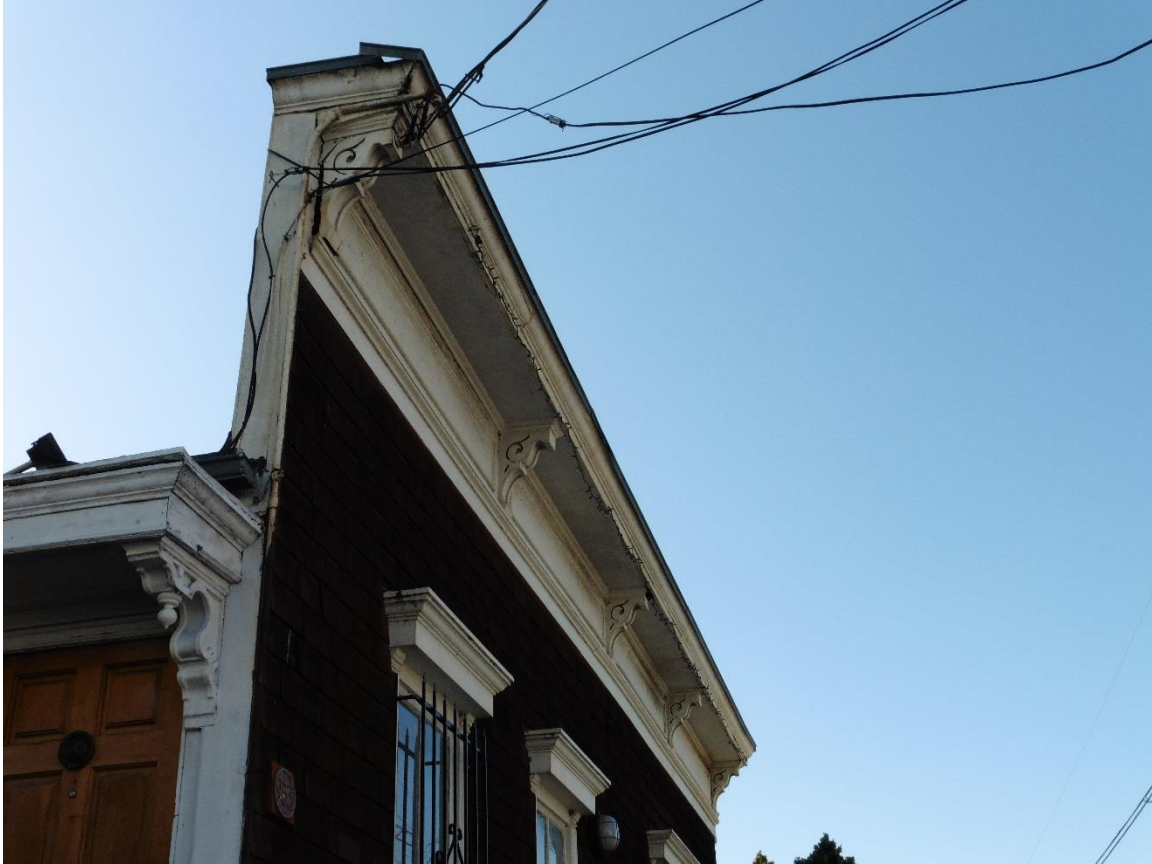
Figure 7. False front and bracketed cornice, looking south along Treat Avenue.
