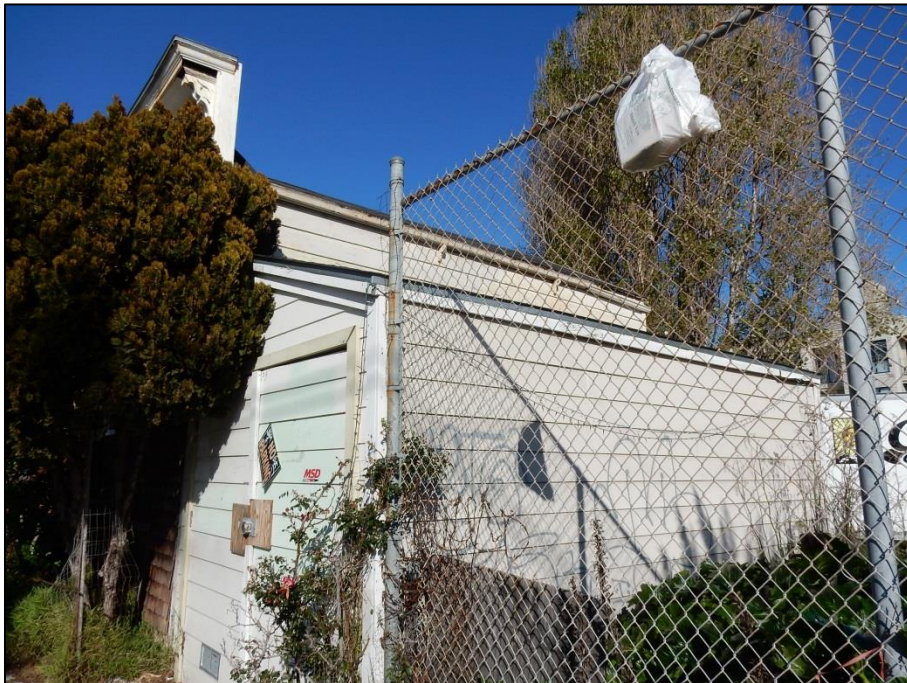
Figure 4 – 953 Treat Avenue – West (left) and South (right) elevation showing shed addition.
