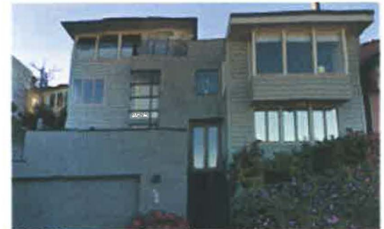
Lot 38 home broken into two parts
