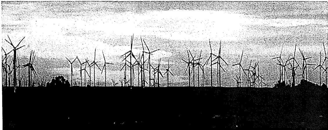
Photo 9: Shiloh I Wind Farm
