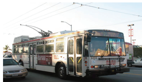
Extension of overhead wire system enables zero-emission transit service to Mission Bay.
