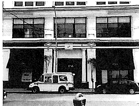
Detail of storefronts. 103_4095.JPG 3/8/2011
