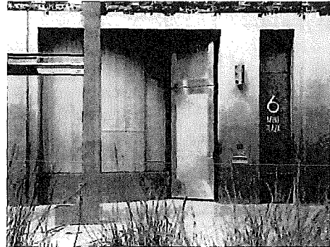
Detail of primary entrance. 103_4044.JPG 3/8/2011
