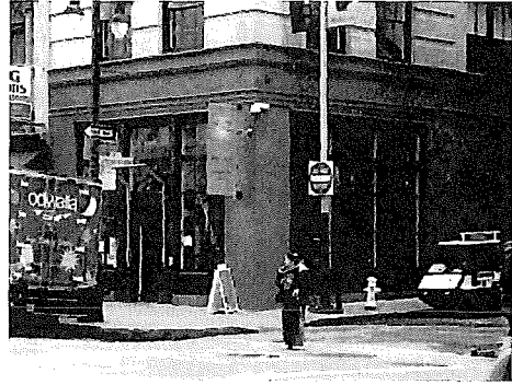
First story storefront. 103_4036.JPG. 3/8/2011
