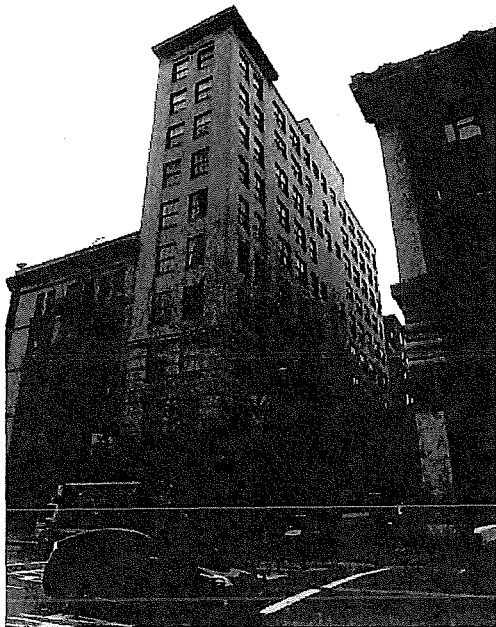
View of northeast and northwest facades. 103_4035.JPG 3/8/2011
