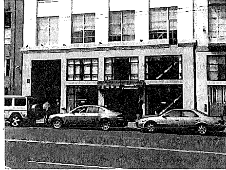
Detail of first story storefronts. 103_4083.JPG 3/8/2011
