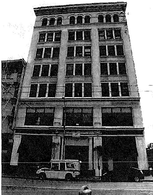
View of northwest facade. 103_4094.JPG, 3/8/2011
