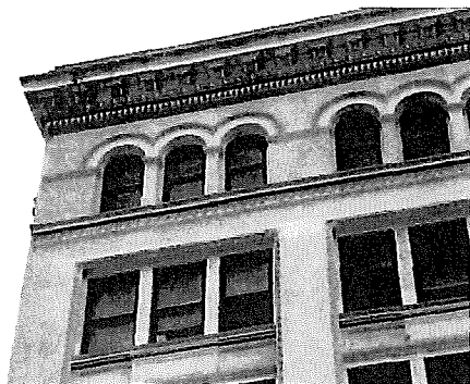
Detail of upper facade. 3/8/2011. 103_4096. JPG
