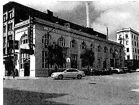
View of southeast and northeast facade. 103_4068.JPG 3/8/2011
