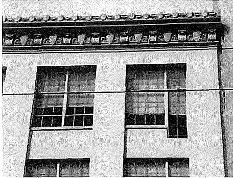
Detail of upper facade and cornice. 103_4082.JPG 3/8/2011
