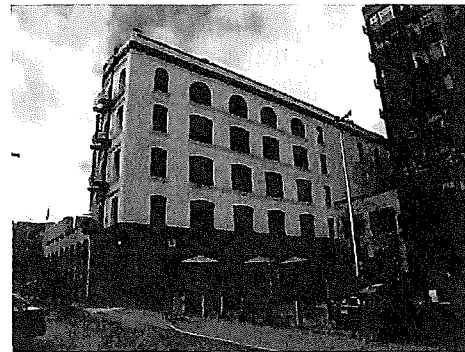
View of northeast facade. 103_4050.JPG 3/3/2011
