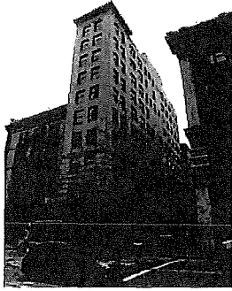
Fifth/Stevensen Street corner view, looking south. 103_4035.JPG. 3/8/2011
