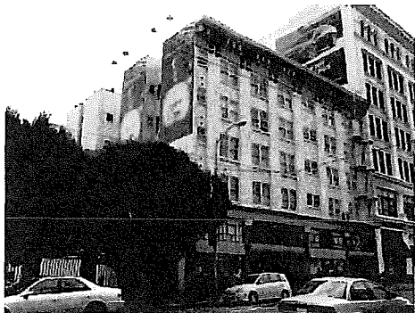
View of northeast and northwest facades. 103_4099.JPG 3/8/2011
