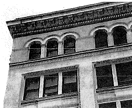
Detail of upper facade. 103_4096.JPG 3/8/2011
