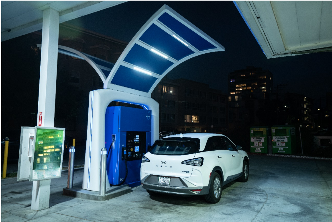
Figure 3 – True Zero Hydrogen Refueling Station
