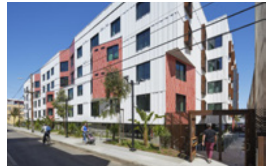
La Fenix affordable housing development (photo: Bruce Damonte)
