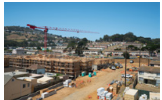
Construction at Sunnydale HOPE SF site (photo: MOHCD)
