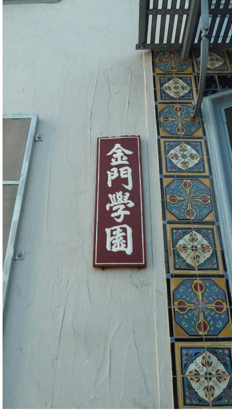
Japanese sign reading "Kinmon Gakuen" to left of main entry door, view south.
