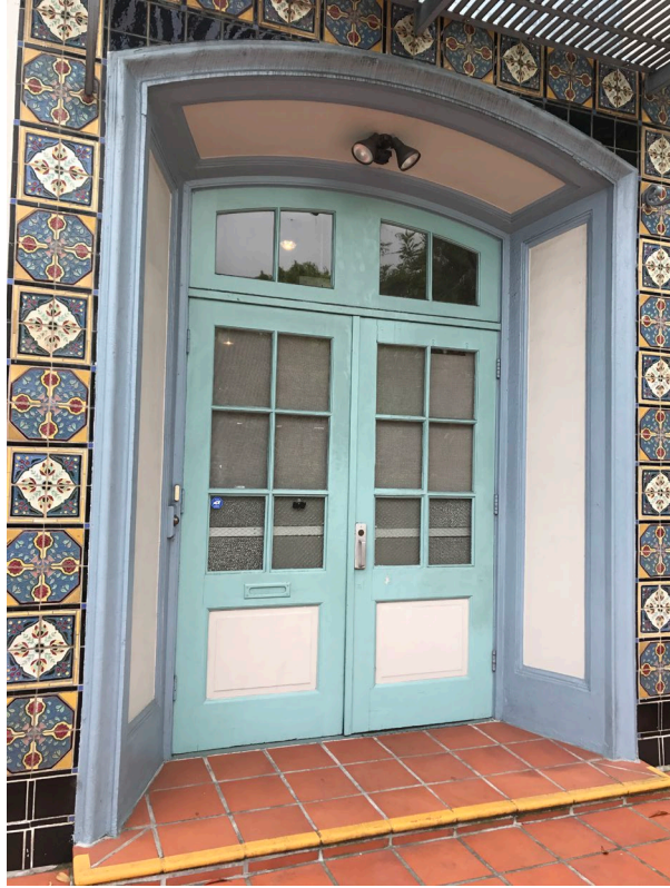
Main entrance, view southwest.
