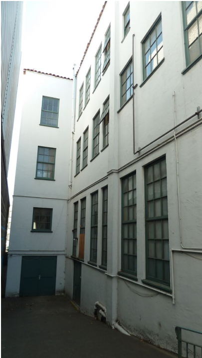
East elevation, view southeast.
