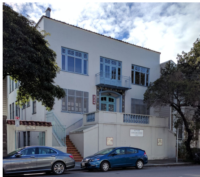
The Kinmon Gakuen Building, 2018.
