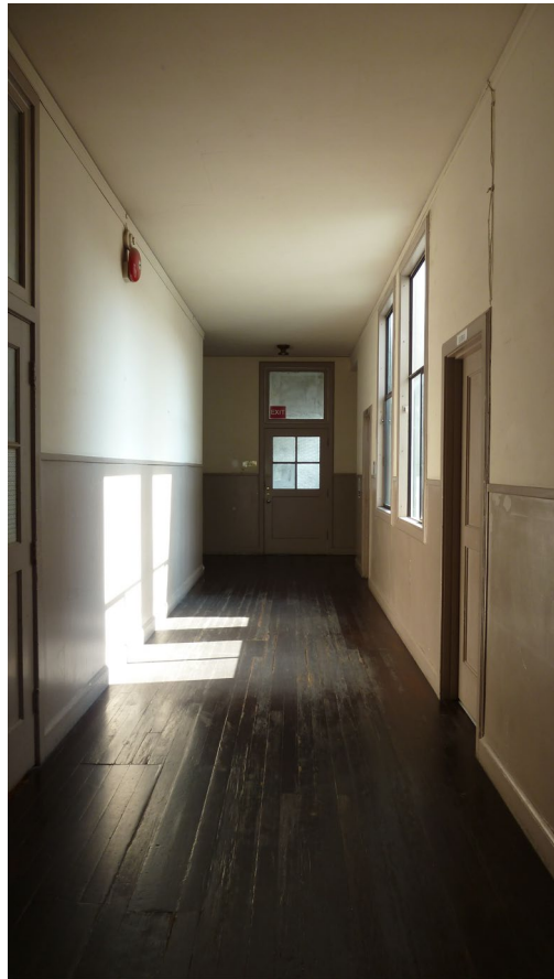
Double loaded corridor leading to classrooms.
