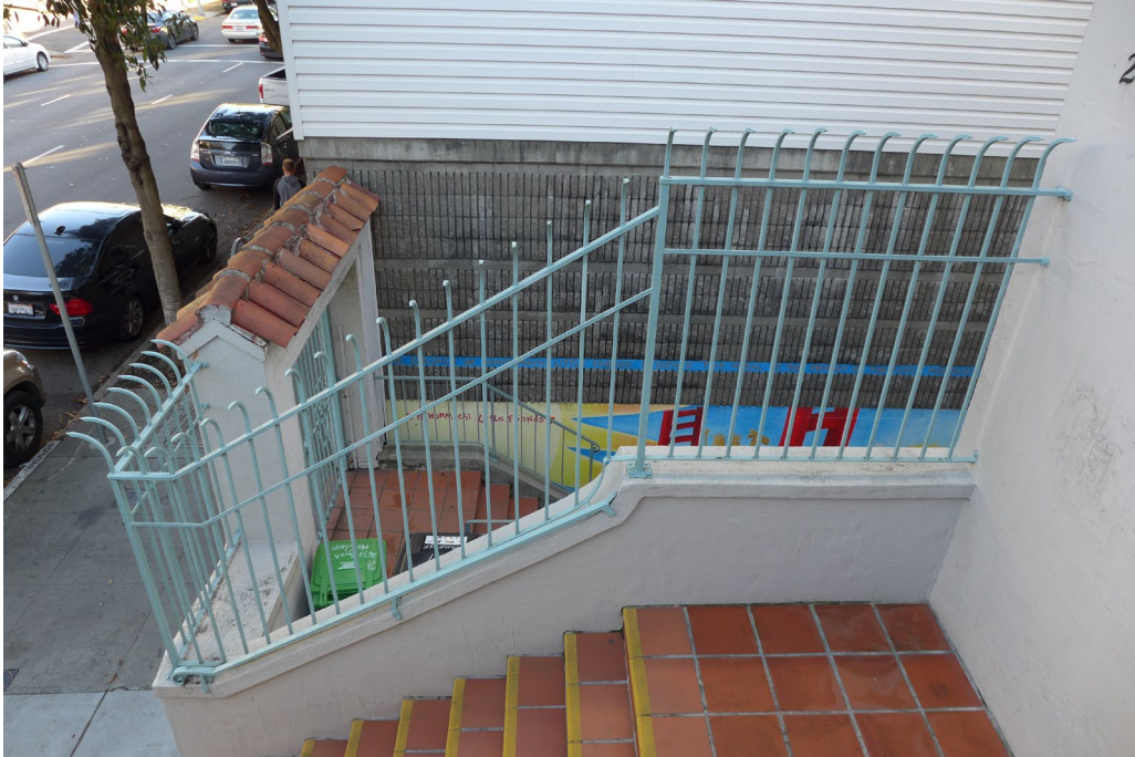
Entry stairs and entrance to side yard, view east.
