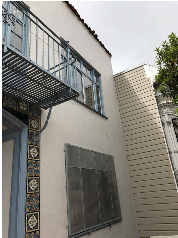
Detail at front façade, view southwest.
