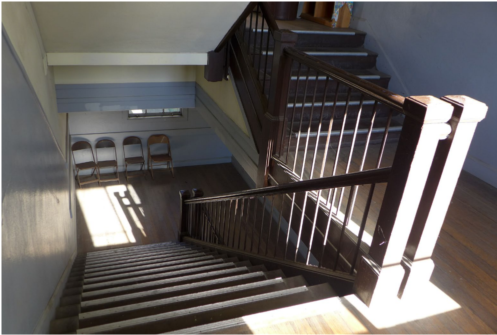
Dogleg, closed string wooden stairs with railing.
