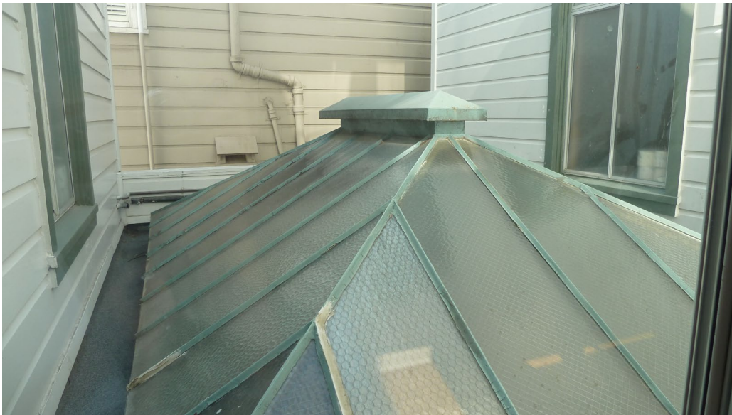
Skylight in light well at west elevation.
