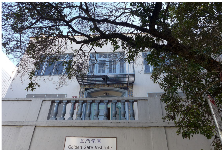
Primary (north) façade, view south.
