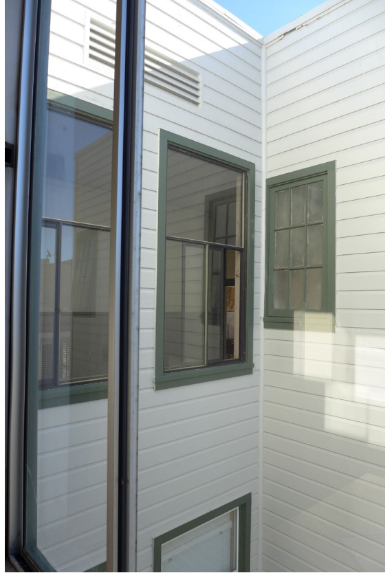
Light well at west elevation.
