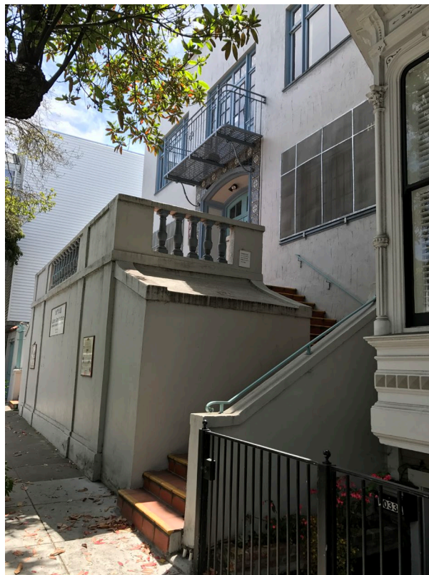
Front façade, view southeast.
