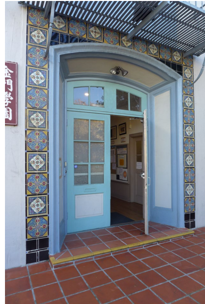
Detail of main entry at front (north) façade, view south.
