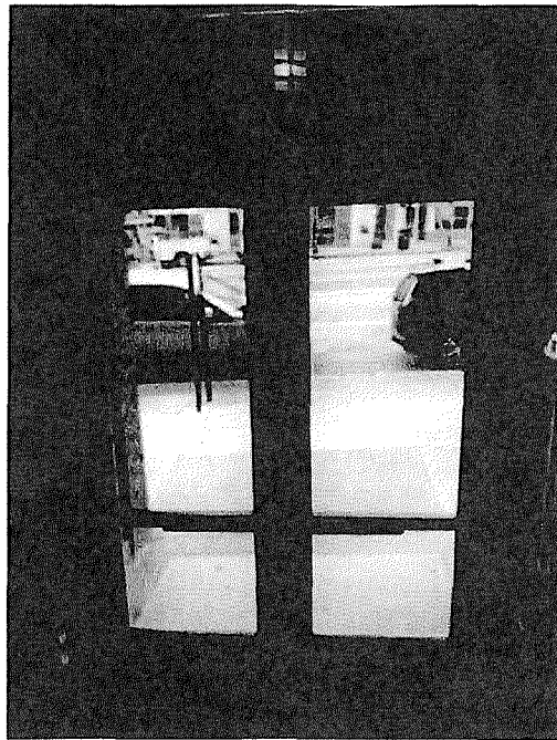
Interior of doors to be replaced.
