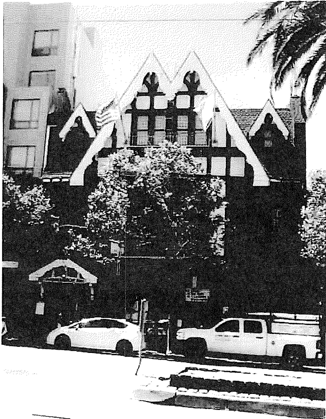
Subject 2168-2174 Market Street
