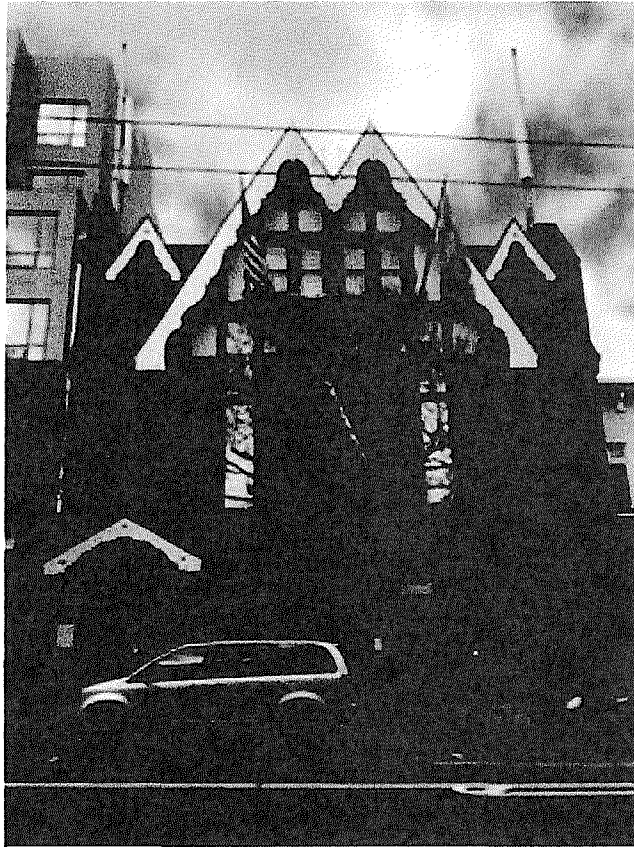
Front building exposure from Market Street.
