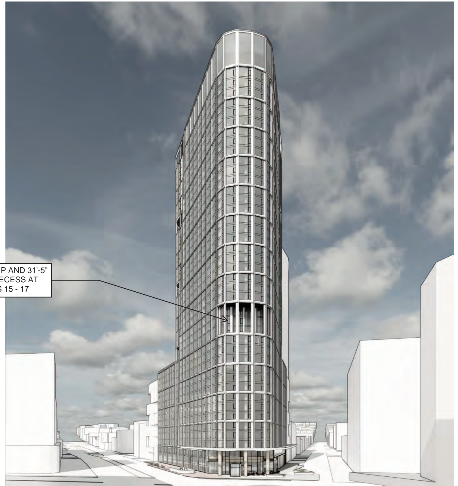
VIEW ON CURB OF MARKET ST.
