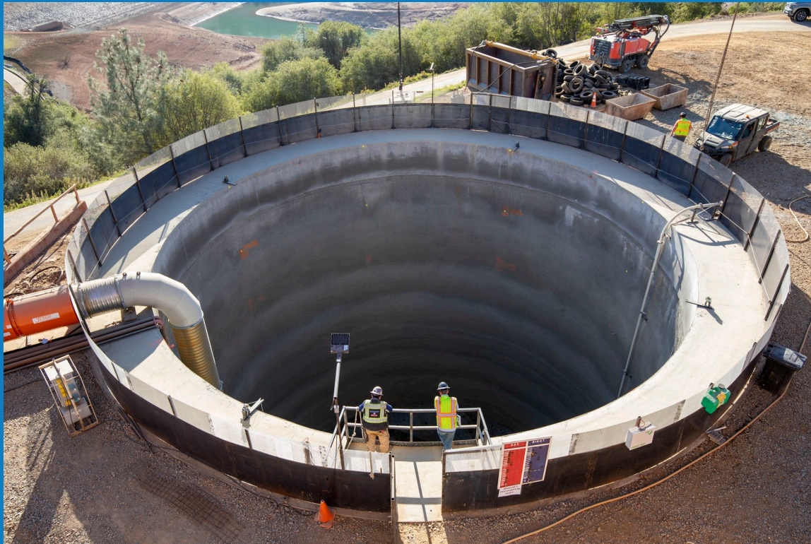
Flow Control Facility Shaft Under Construction
