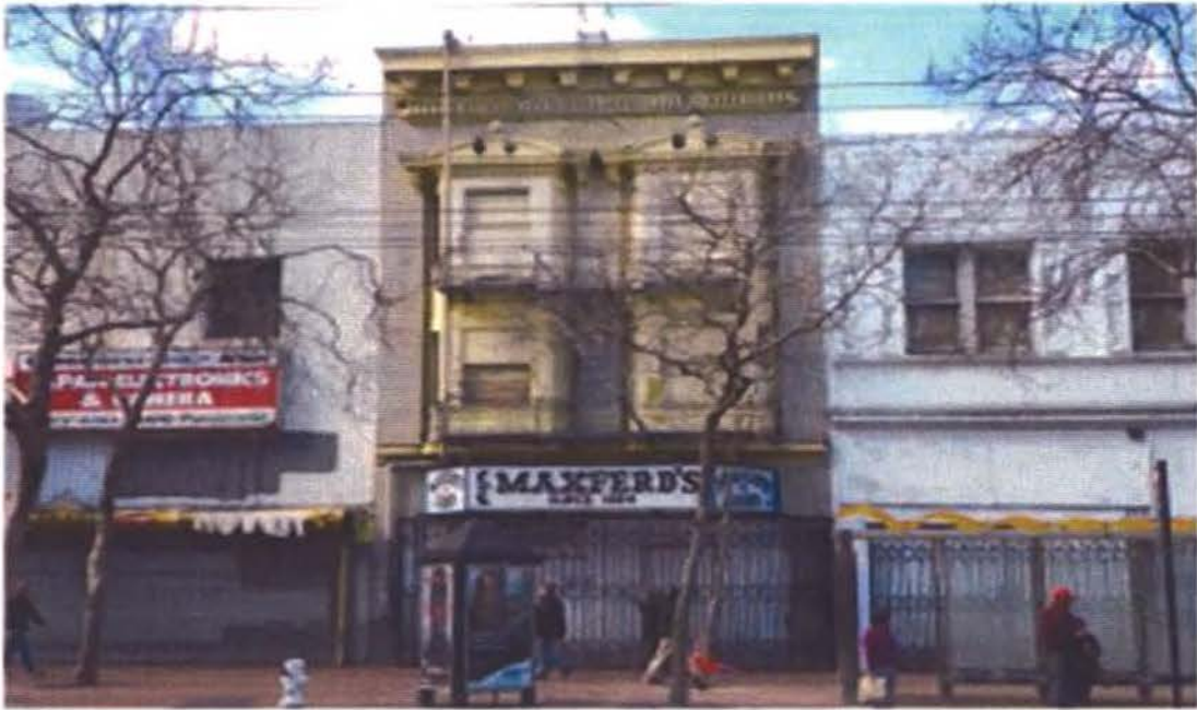
Figure 23. 972 Market Street, primary (southeast) facade.
