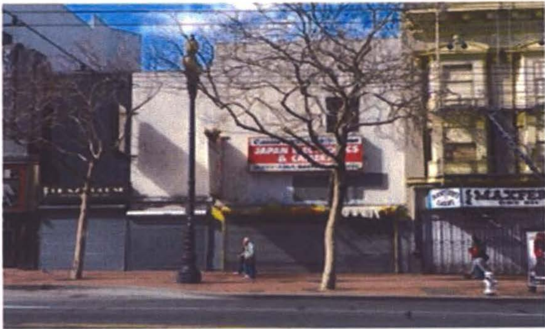
Figure 26. 974 Market Street Southeast Facade (Tim Kelley Consulting, March 2011)
