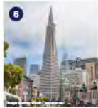
6 Transamerica Pyramid 600 Montgomery Street Year Built: 1976 Significant for its Brutalist architecture designed by architect of merit William Pereira & Associates
