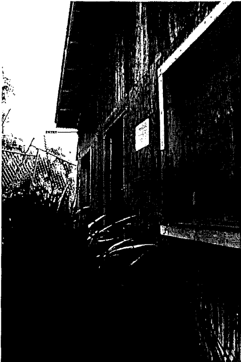
4 COTTAGE: EXISTING NORTH FACADE NOT TO SCALE
