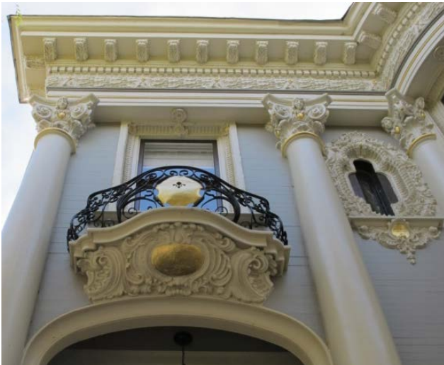
Figure 16: North side of primary façade.
