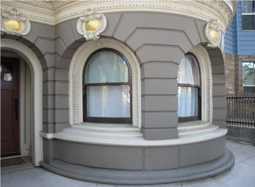
Detail of rusticated base
