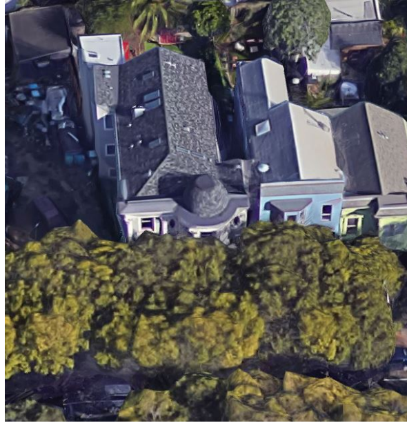
Figure 21: Aerial photograph from Google Maps, 2016.
