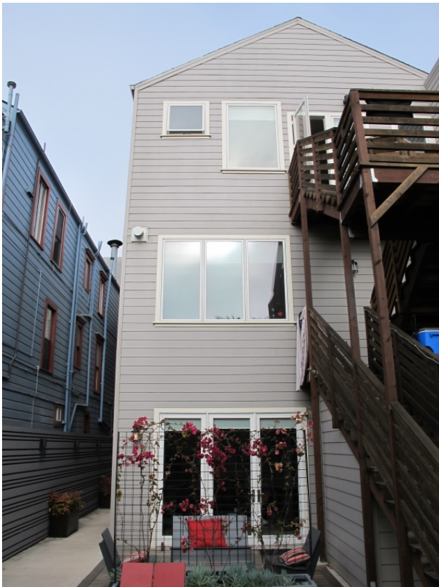
Figure 29: South side fenestration.
