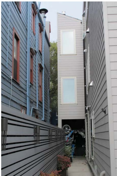
Figure 22: South façade with projection and passageway, view facing west.
