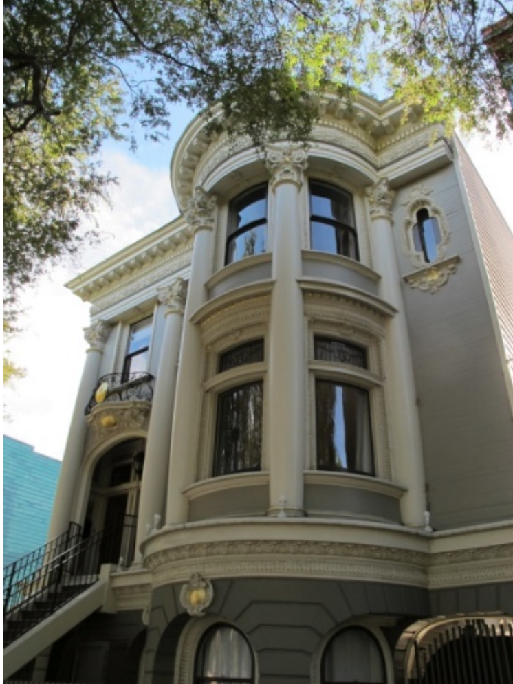
Figure 4: Ground level of primary façade.
