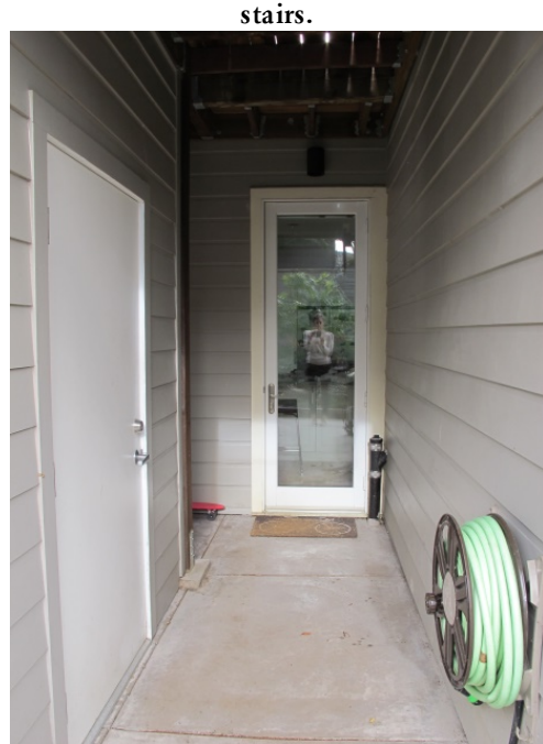
Figure 28: Storage door and south façade access door.
