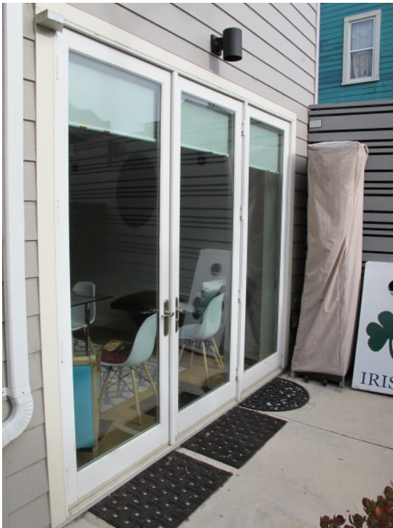
Figure 31: North side ground level.
