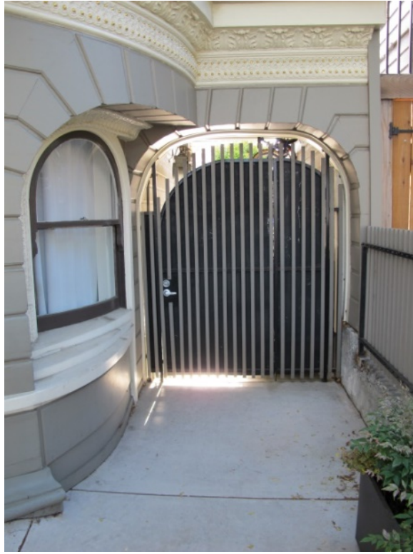
Figure 8: Security gate leading to south façade and backyard.
