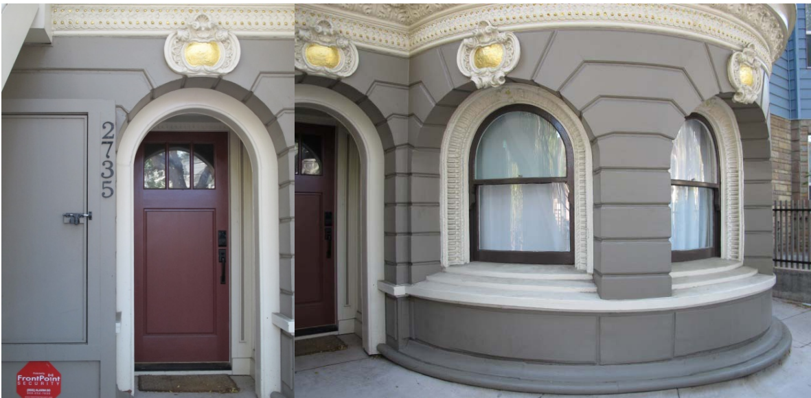
Figure 5: Entry to Unit 2735.
