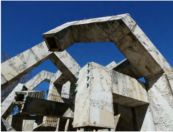
Overall view and condition of hollow, pre-cast concrete arms of fountain, looking north.
