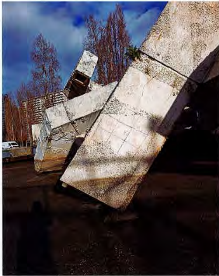
Photo 1. Side view of one of the tubes with GPR scan markings on the face of the tube.
