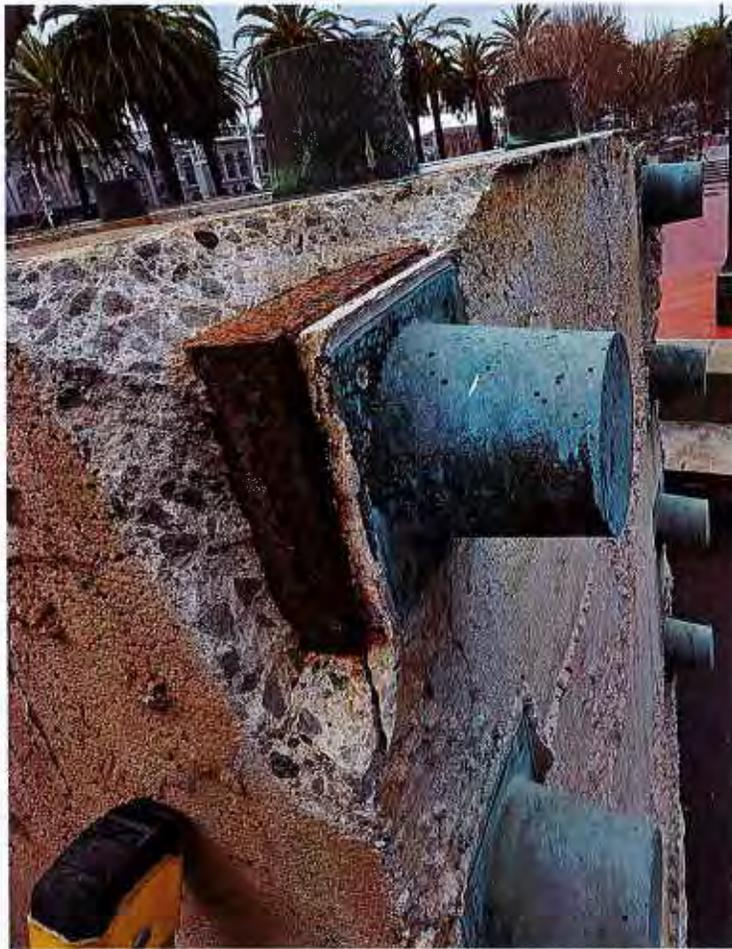
**Photo 3. Steel plate at end cap.**
