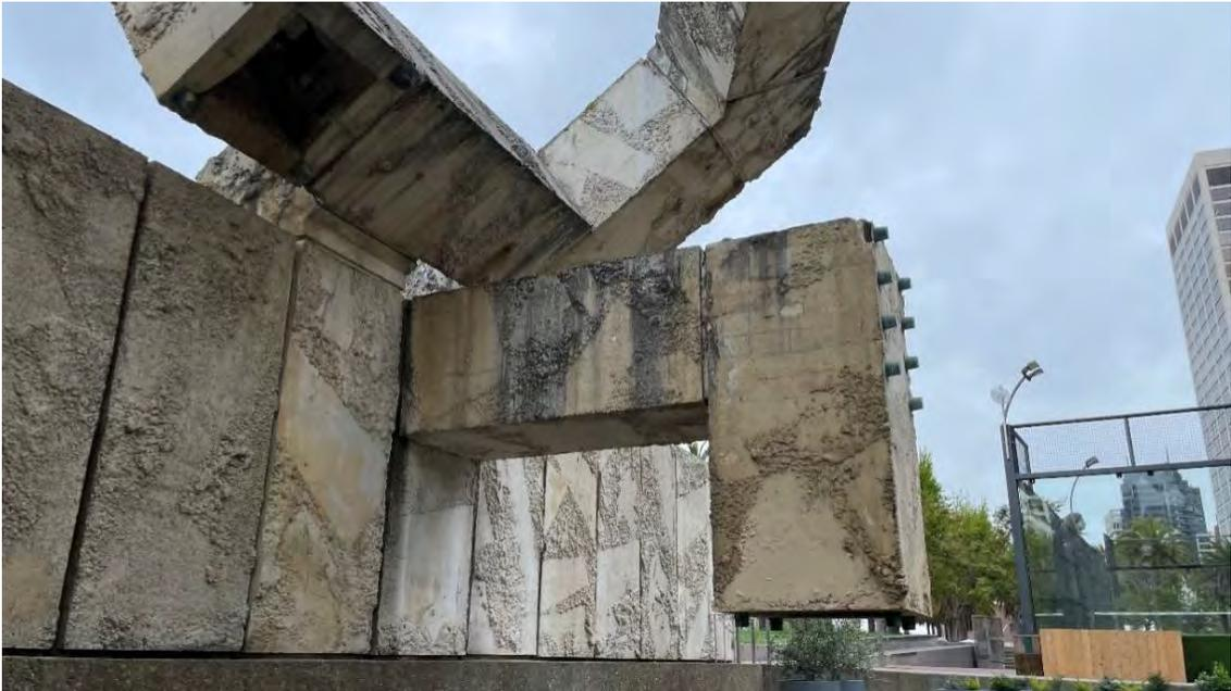
*Figure 5: Vaillancourt Fountain - Cantilevered Elements Showing Tension Rods and Caps*
