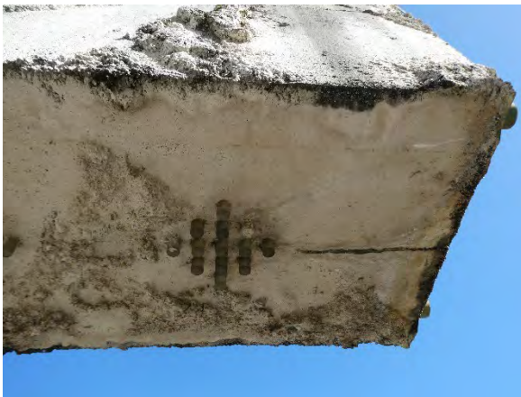
Detail of glass cylinders in the hollow pre-cast concrete arms, associated cracking, and efflorescence.
