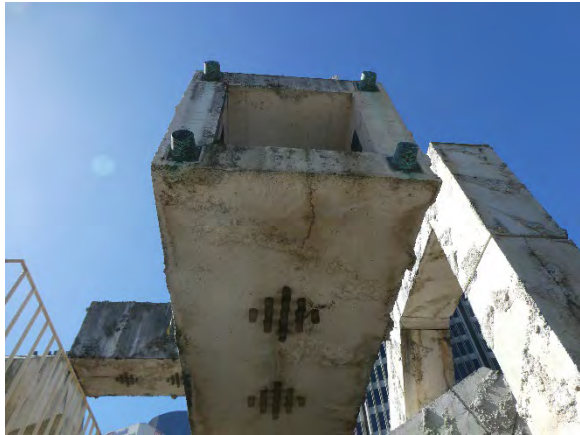
Central crack at lower side of projecting column, typical condition. Northeast elevation pictured.
