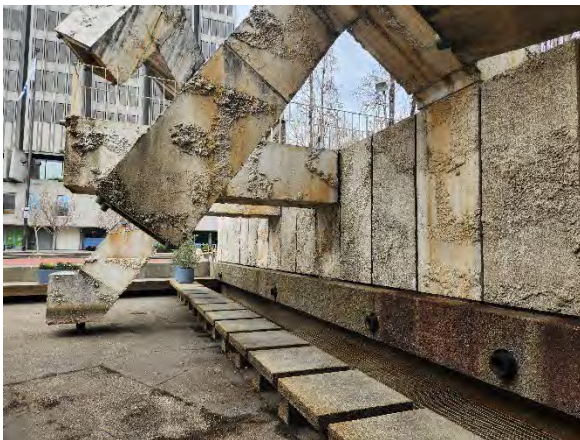
Typical overall condition of concrete “lily pad” pedestals, north side of fountain, looking west.
