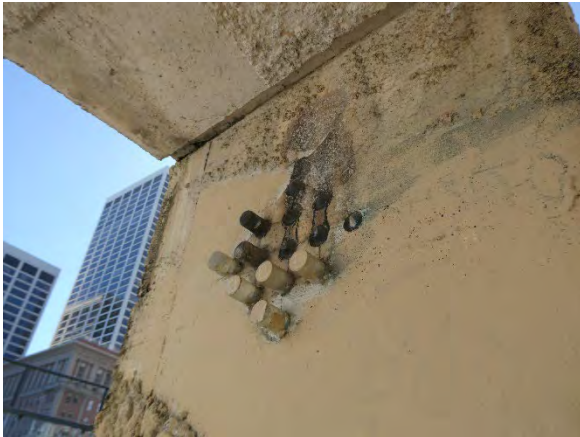
Detail of broken and painted glass cylinders in the hollow pre-cast concrete arms.
