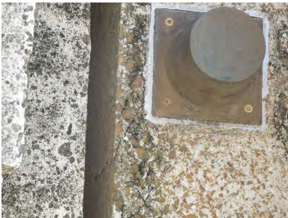
Incipient spalling adjacent to metal fixture, typical condition. Northeast elevation pictured.
