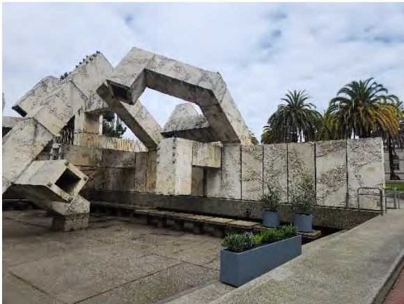
Overall view of the hollow, pre-cast concrete panel wall, east side of fountain looking northeast.
