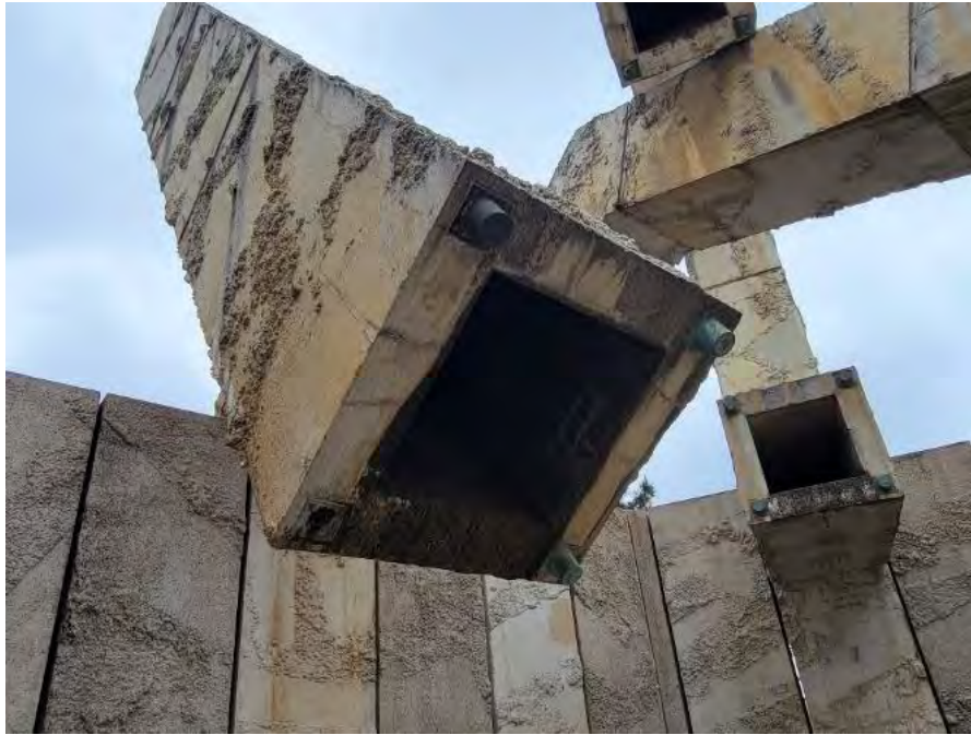
Figure 11: Vaillancourt Fountain – Showing Corroded End Plate and Absence of Thru Rod and Spalled Concrete Surface
