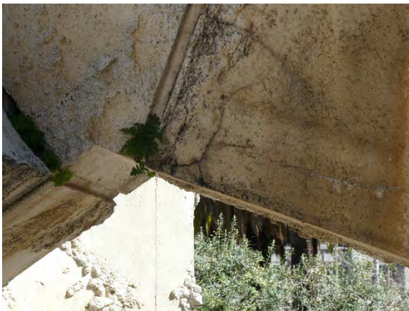
Incipient spalling and cracking at joint of projecting column, typical condition. Biological growth within several cracks.
