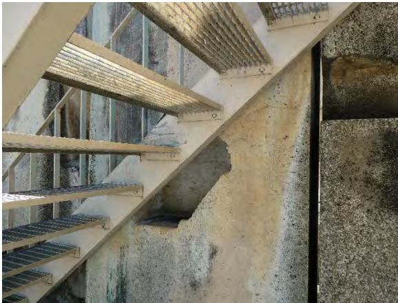
Typical condition of the underside of the painted steel stairs on the east side of the fountain, exhibiting soiling but minimal if any corrosion.
