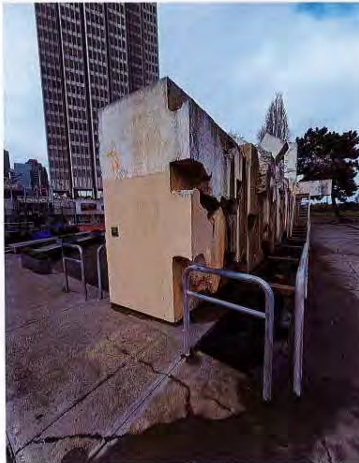
Photo 4. Rear wall – no reinforcing steel was found.
