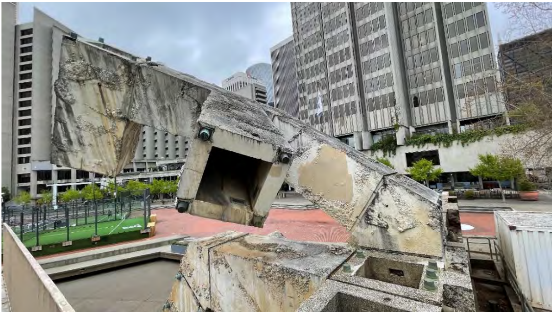
Figure 6: Vaillancourt Fountain - Cantilevered Elements Showing Tension Rods and Caps
