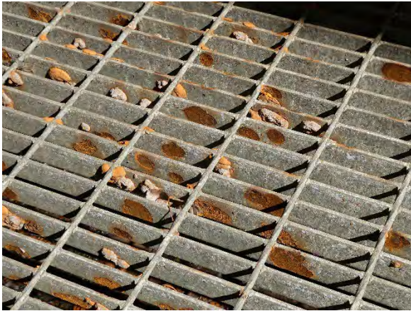
Typical corrosion at metal grate over sump pit.
