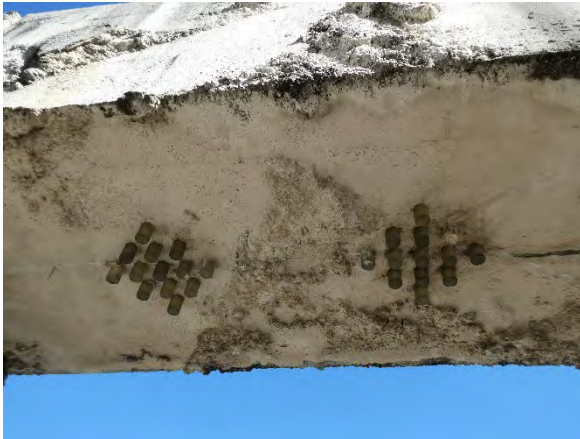
Detail of glass cylinders in the hollow pre-cast concrete arms, associated cracking, and efflorescence.
