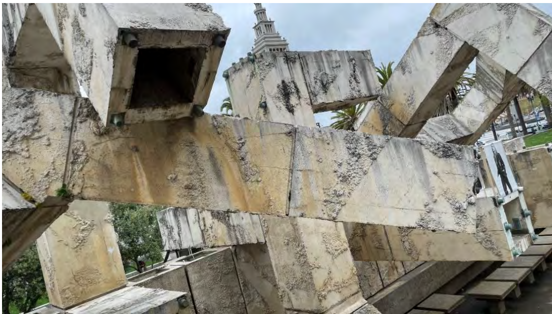
Figure 14: Vaillancourt Fountain – TS6 Frame resting on TS4-TS5 Assembly with Cracks and Corrosion Close Up
