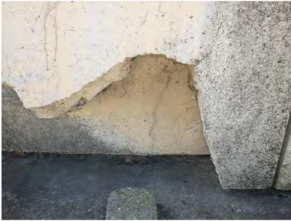
Cracks at base, typical condition. Northeast elevation pictured.
