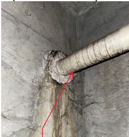
This is the only area where ACM pipe insulation was identified. This insulated pipe run exits the room through a wall opening, presumably to the exterior underground area)
