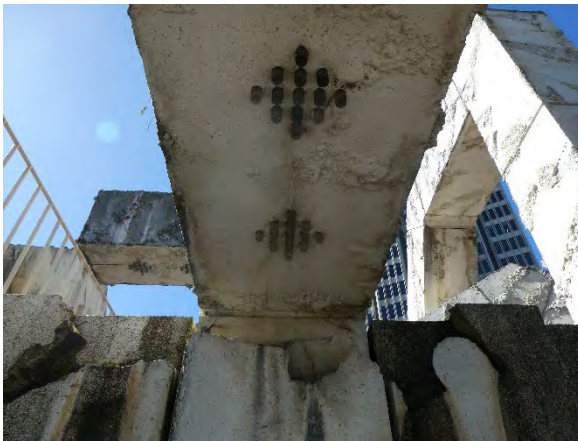
Typical glass cylinders on the underside of the hollow, pre-cast concrete arms.
