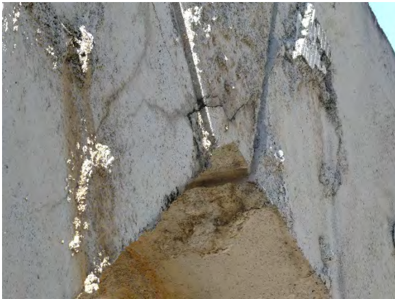
Incipient spall and cracking at joint of projecting column, typical condition.
