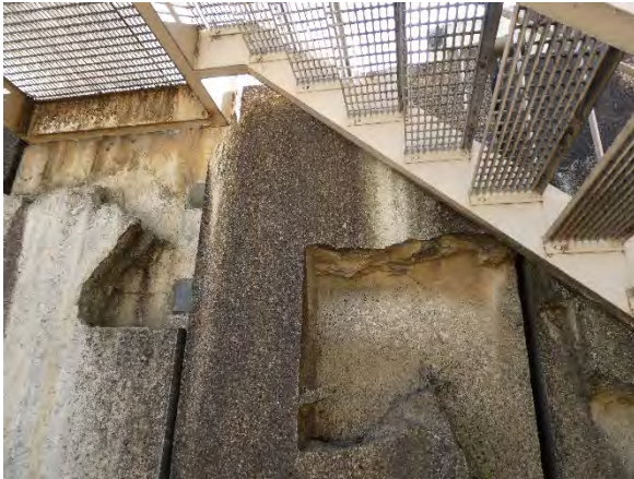
Typical condition of the painted steel stairs with soiling, and some minor surface corrosion at edges of the landing frame.
