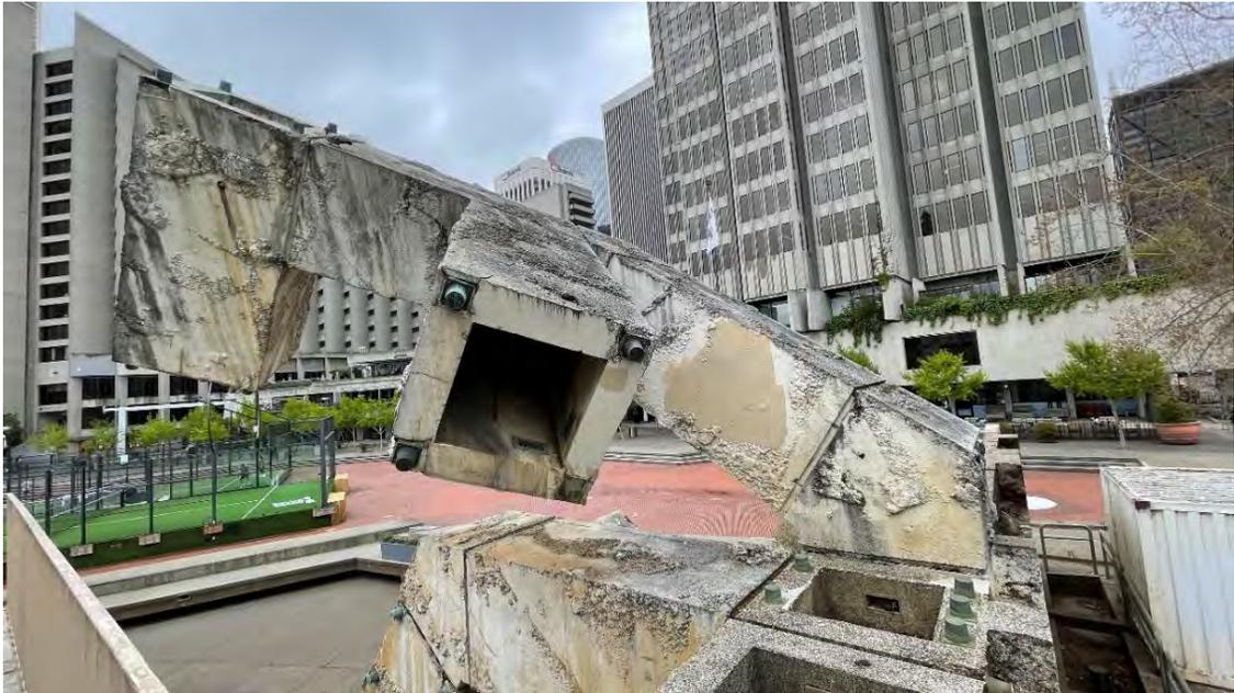
*Figure 6: Vaillancourt Fountain - Cantilevered Elements Showing Tension Rods and Caps*
