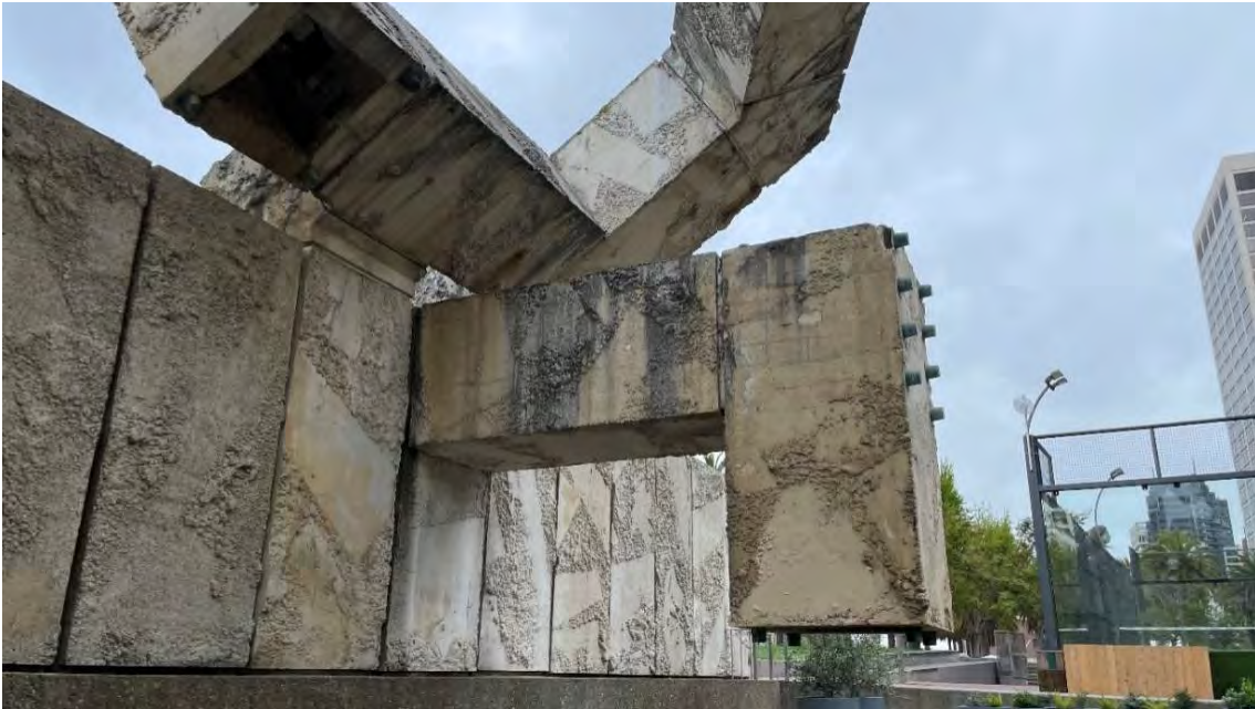
Figure 5: Vaillancourt Fountain - Cantilevered Elements Showing Tension Rods and Caps
