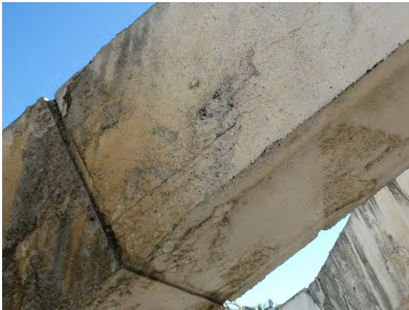
Cracking at the joint along the underside and side of projecting column, typical condition.
