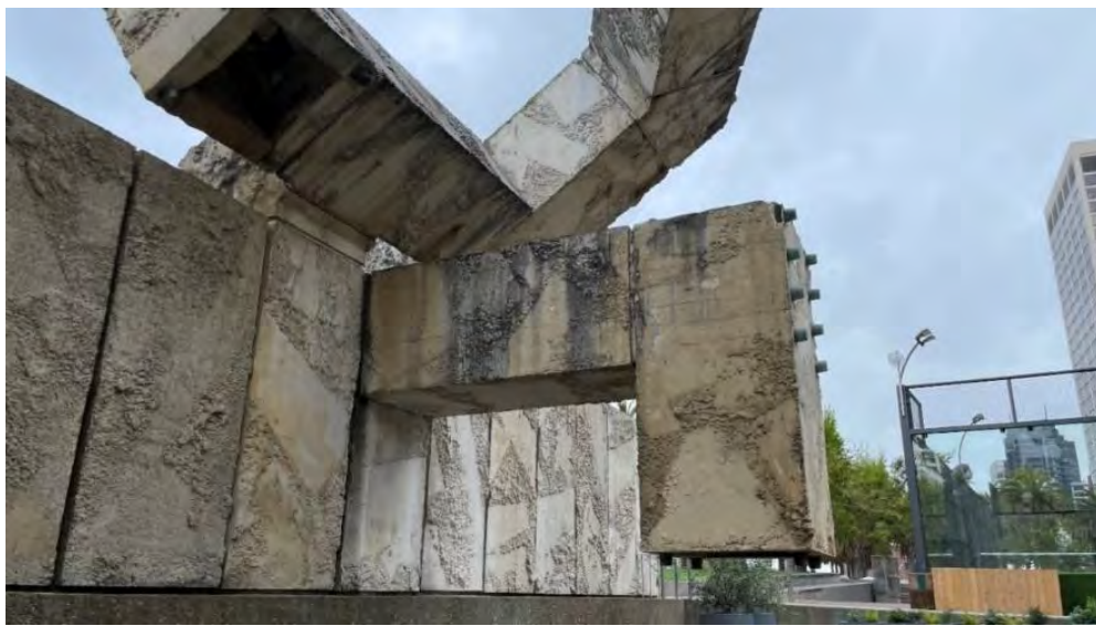
Figure 9: Vaillancourt Fountain - Showing Spalled Ends
