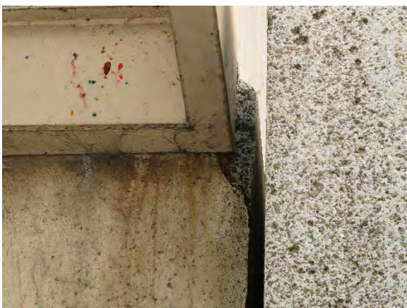
Incipient spalling at the joint beneath metal stair platform, typical condition. Northeast elevation pictured.
