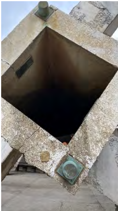
Figure 12: Vaillancourt Fountain Cracked and Spalled Concrete and Water Damage Stains
