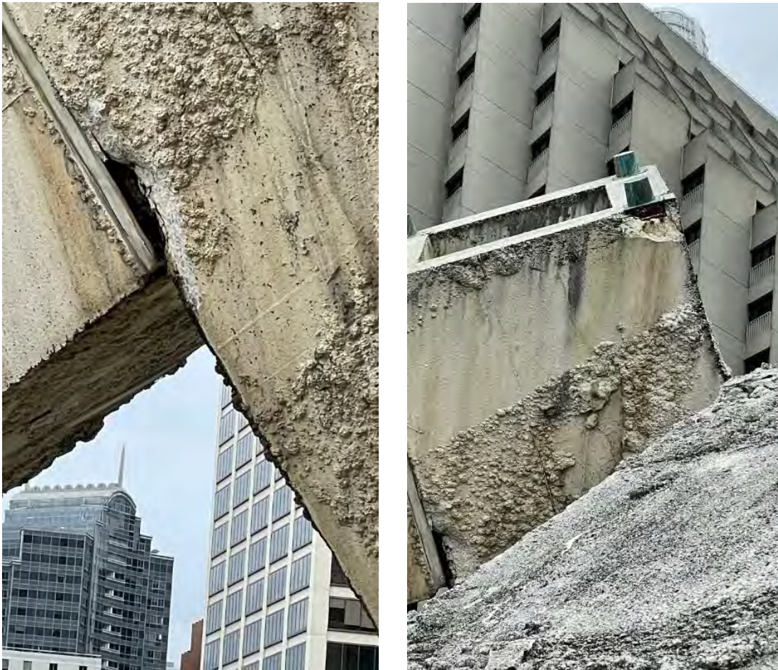
Figure 10: Vaillancourt Fountain - Spalled and Cracked Concrete and Corrosion of Steel Elements
