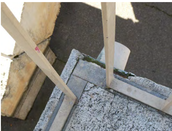
Detail of spalled concrete at the edge of the railing attachment.
