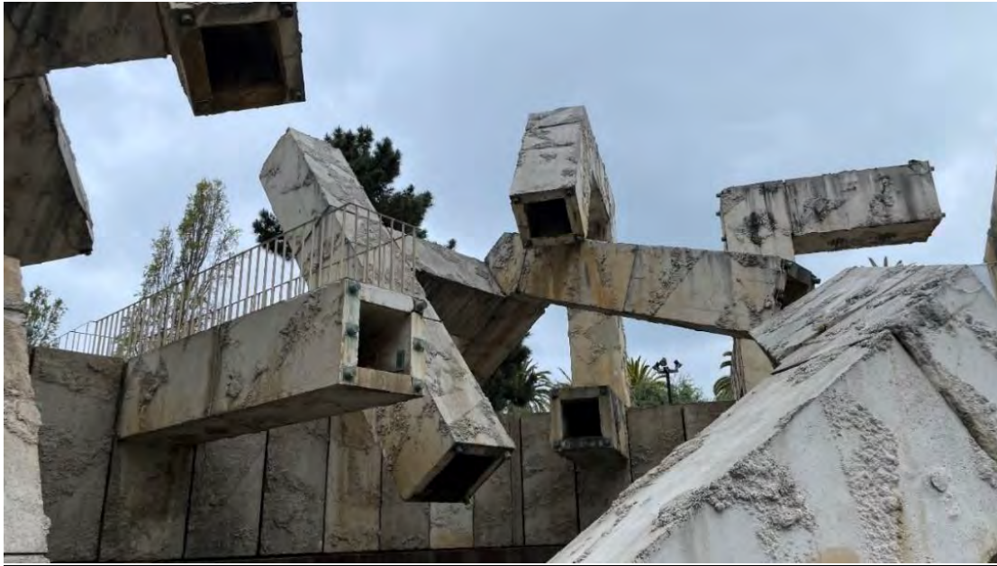
Figure 13: Vaillancourt Fountain – TS6 Frame on TS4-TS5 Assembly - Cracks and Corrosion
