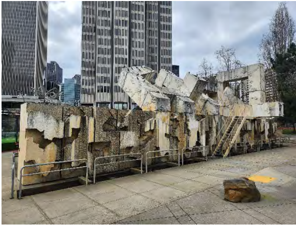
Overall view of the hollow, pre-cast concrete panel wall, east side of fountain looking northwest.
