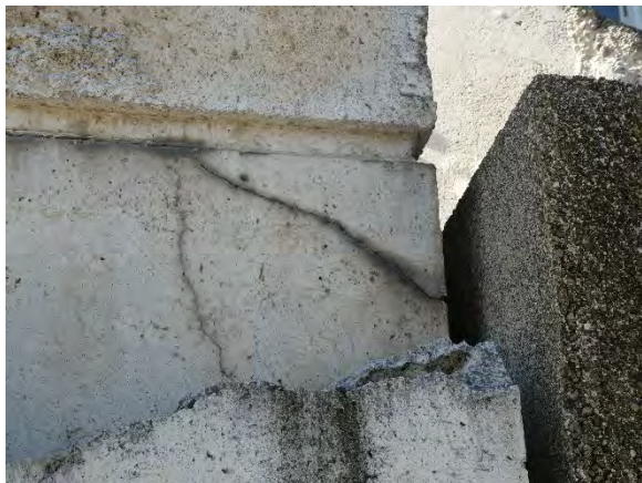
Incipient spalling and cracking at joint of vertical column, typical condition. Northeast elevation pictured.
