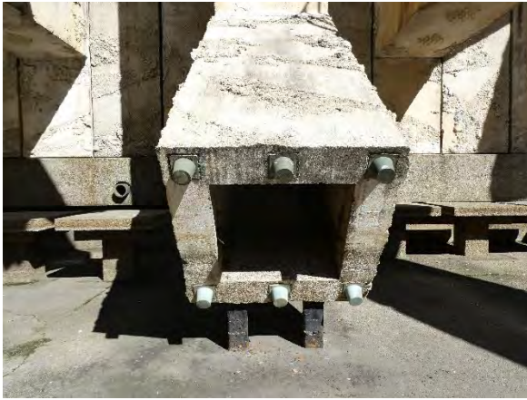
Typical condition of concrete pool and connections between concrete pool and hollow pre-cast concrete “arms,” showing cracking, biological growth, soiling, and corrosion at connections.
