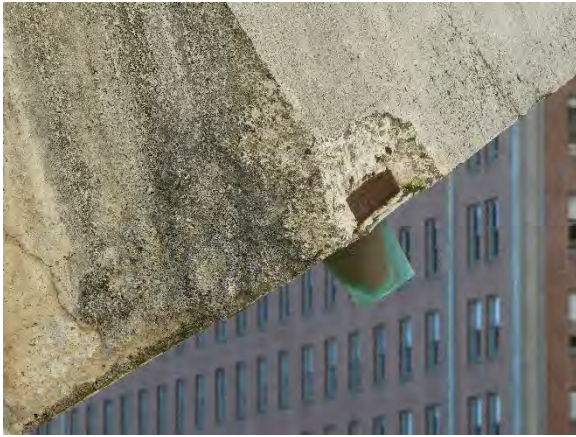
Spalling at the outer corners of the projecting column, typical condition. Image taken facing south.
