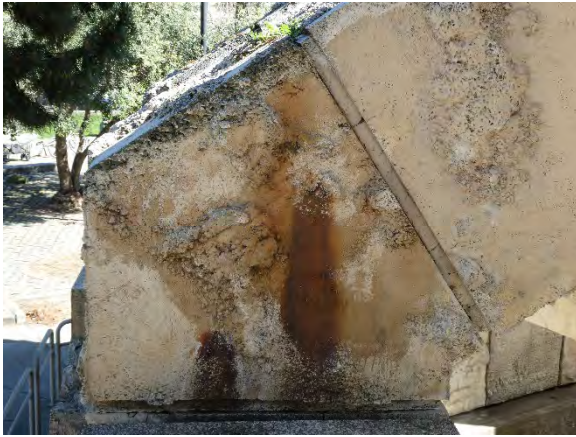
Corrosion of metal fixtures, typical condition. Photo facing west from viewing platform.
