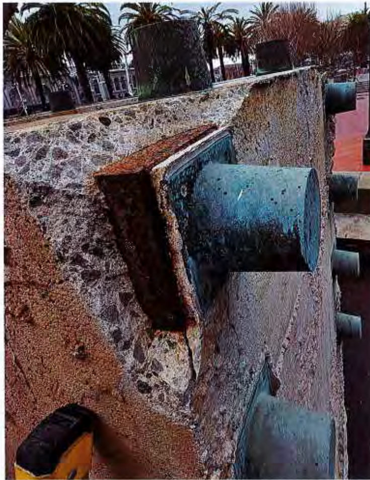
Photo 3. Steel plate at end cap.
