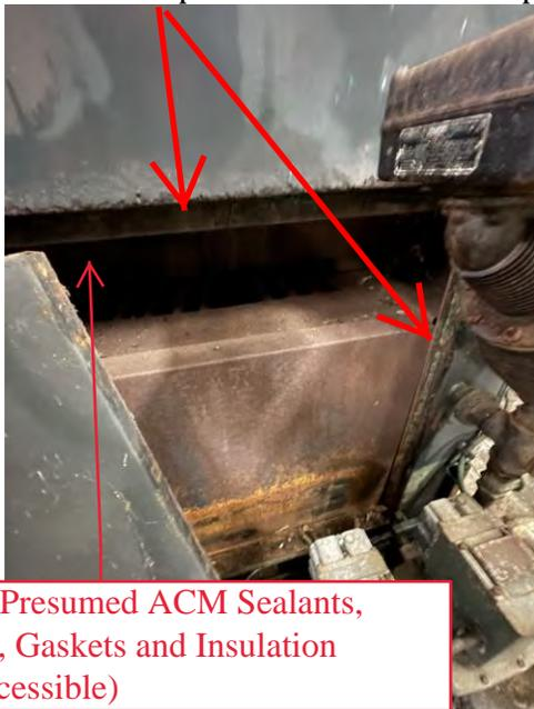
Boiler Interior is Presumed ACM Sealants, Ribbing Material, Gaskets and Insulation (Concealed/ Inaccessible)
