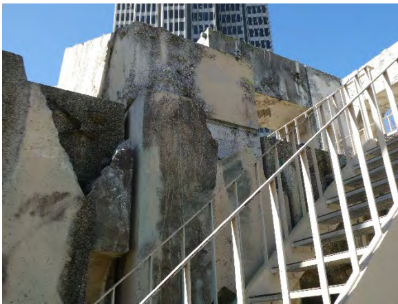
Typical overall condition of painted steel stairs on the east side of the fountain.
