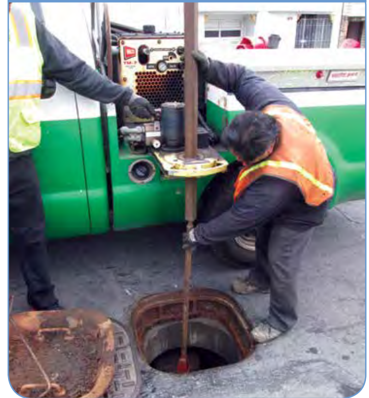
Clear space around water valves is necessary to access, operate, and maintain the valves.
