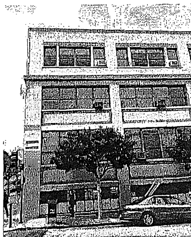
FRAME AND INFILL WITHIN DISTRICT 300 Broadway
