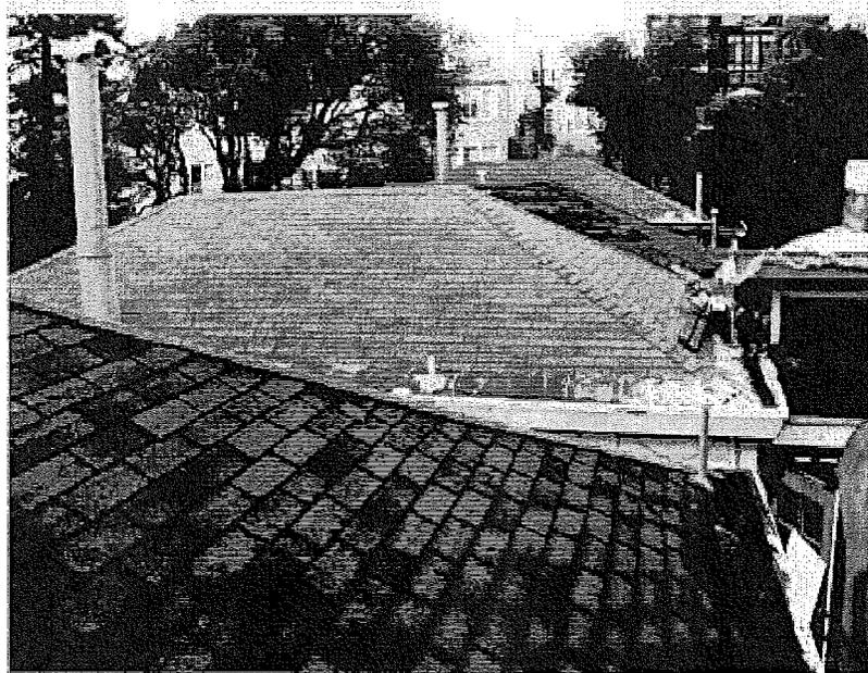
Figure 5. Detail of cottage roofs. Note the round metal flues on the cottages.
