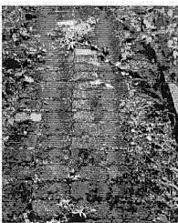
Figure 4: Walkway showing "stacked" coursing and raised brick planter
