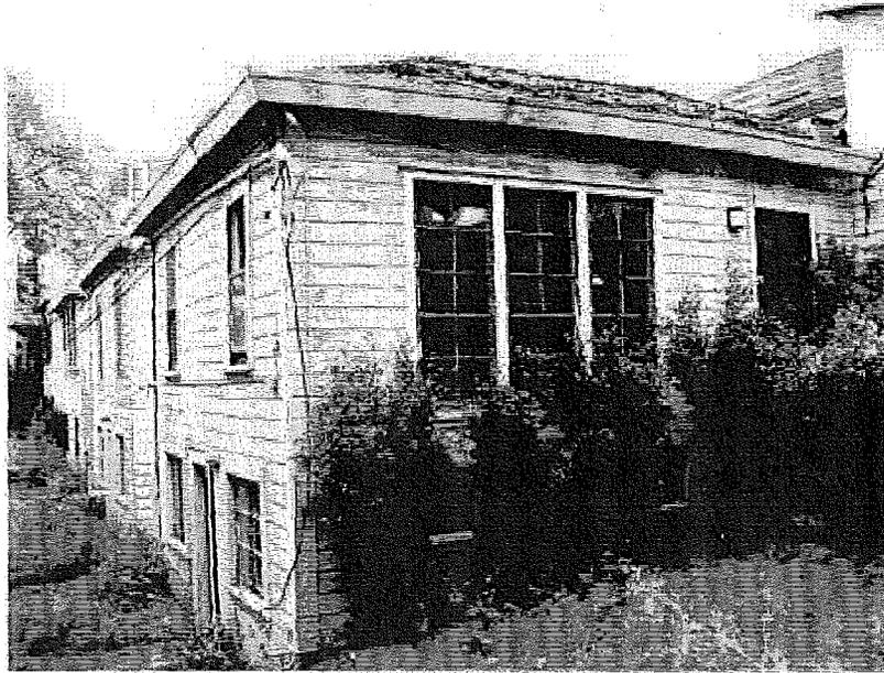
Figure 3: View of the primary (west) facades of the cottages and south façade of Cottage A. Note boxed eaves.
