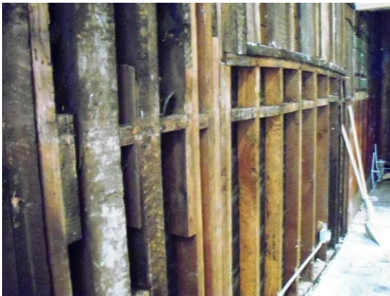
Interior of exterior wall along Emery Lane
