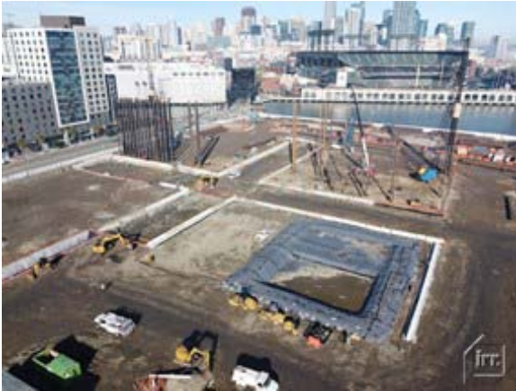
Aerial – Facing North
