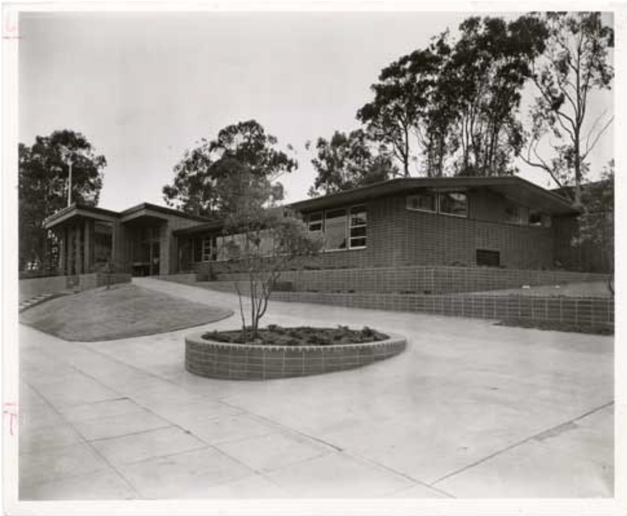
Parkside Branch Library, view northwest, June 19, 1951.
