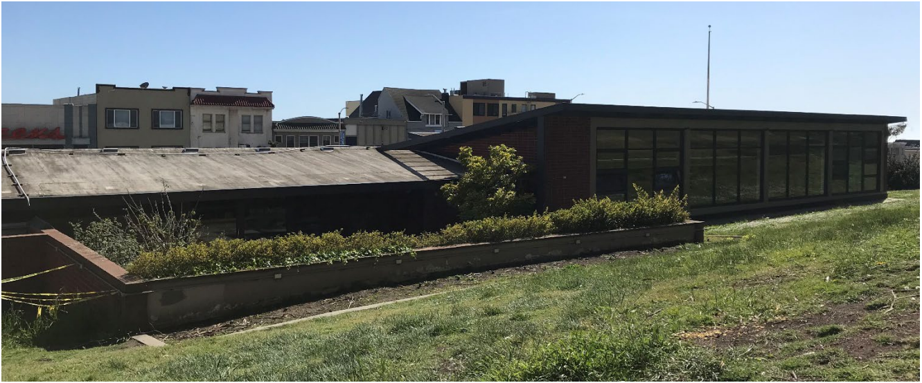
Parkside Branch Library, north elevation, view southwest, 2023. Source: San Francisco Planning Department
