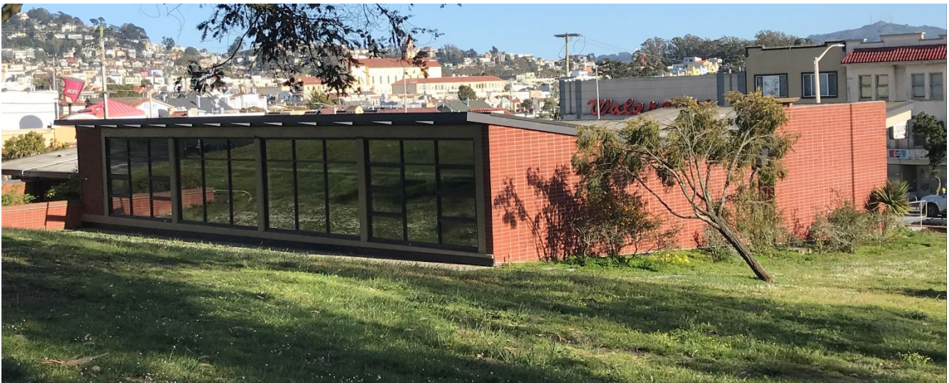
Parkside Branch Library, north elevation, view southeast, 2023. Source: San Francisco Planning Department
