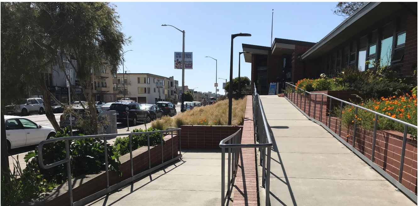
Parkside Branch Library, ramp at front, view west, 2023. Source: San Francisco Planning Department
