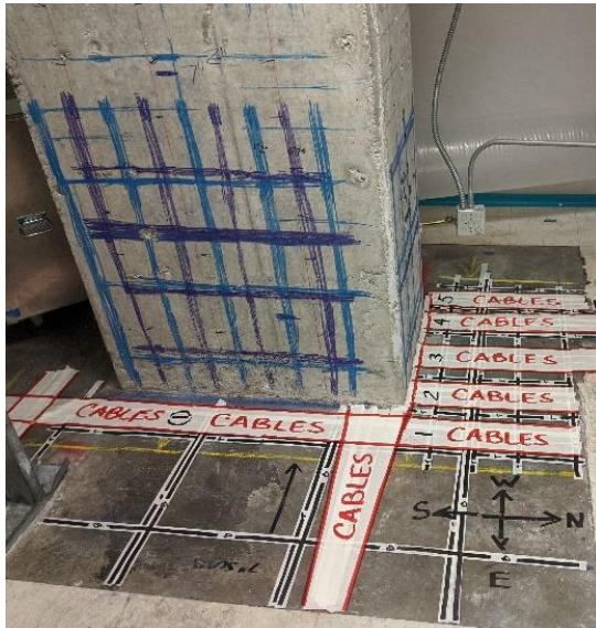
Typical Column Strengthening/Enlargement Process (Scanning, Rebar Installation, and Concrete Placement)
