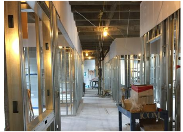
Interior framing and buildout
