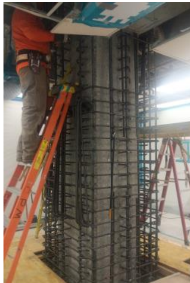
Typical Column Strengthening/Enlargement Process (Scanning, Rebar Installation, and Concrete Placement)
