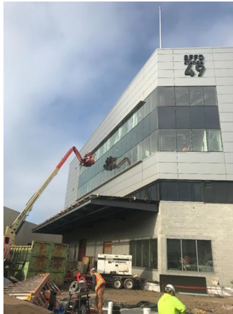
Exterior building façade installation
