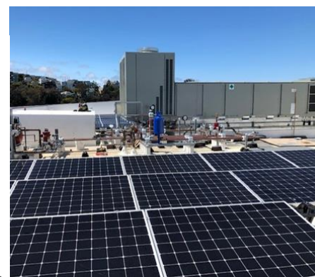
Roof photovoltaic panels
