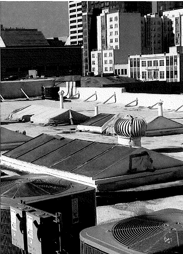
Figure 4. Skylight; note covered ventilation grilles.
