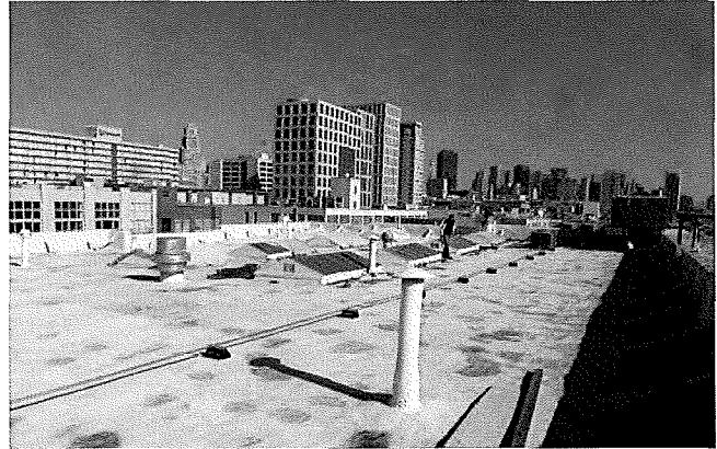
Figure 1. Roof of 149 9th Street, typical.
