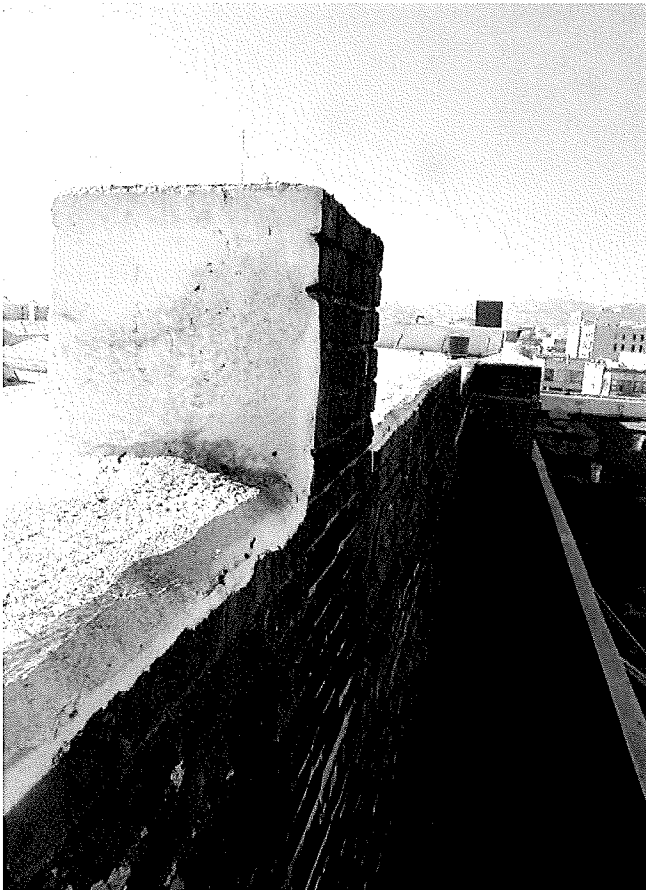
Figure 3. Unbraced ventilation stack at north wall.
