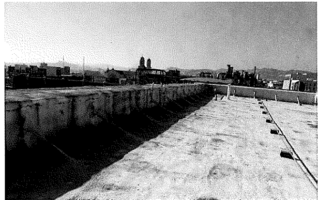
Figure 3. Parapet with bracing, typical.
