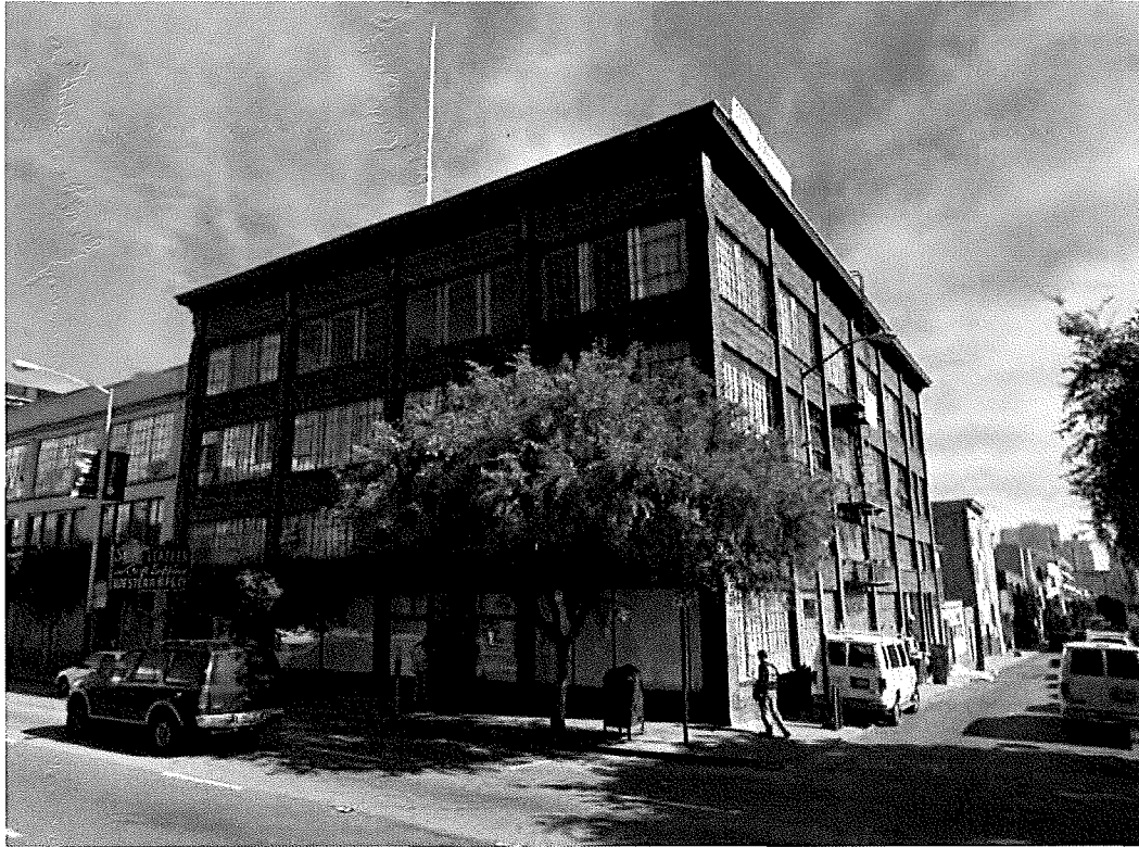
View east of the primary (west) and south facades (Google Maps ©2013)
