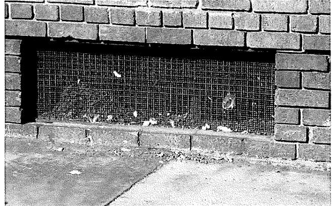
Figure 1. Ventilation grilles; note 1"x1" historic iron grille.
