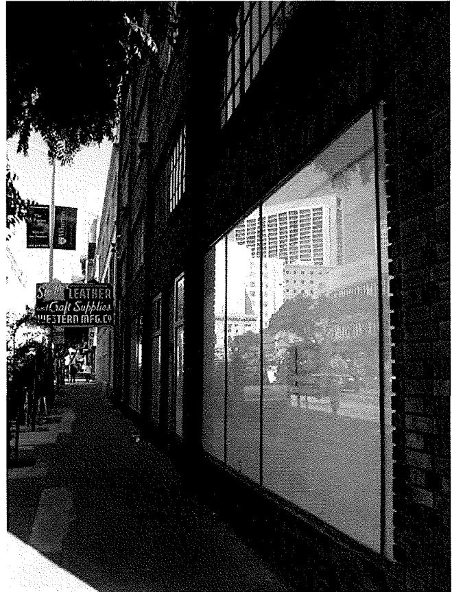
Figure 1. Typical Storefront at west elevation.
