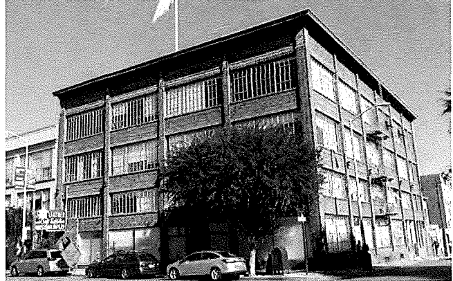
Figure 1. 149 9th Street; view from 9th Street looking east.
