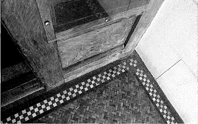
Figure 3: Sidelight at entry door; note replacement of glazing for Plexiglas in response to security concerns.
