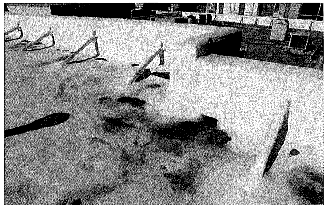
Figure 2. Roof at drainage opening in parapet; note parapet bracing and conditions near opening.
