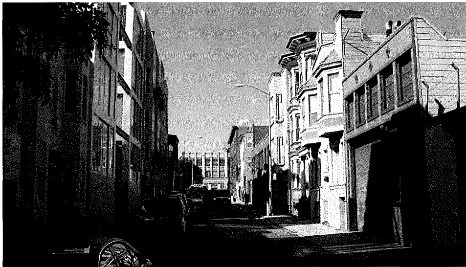
View west along Natoma Street toward the subject building showing a mixture of small scale residences and light industrial buildings. (Google maps, 2013)
