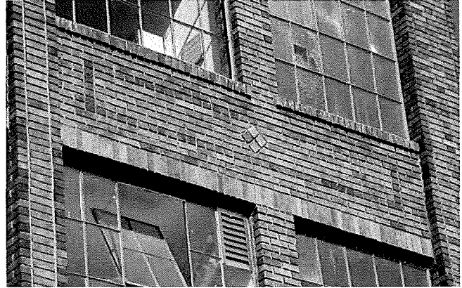
Figure 3. South elevation; note recessed mortar joints to be maintained and replicated in re-pointing.
