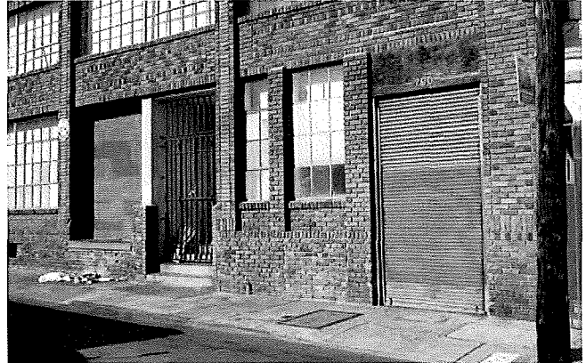
Figure 1. Service doors along south elevation.
