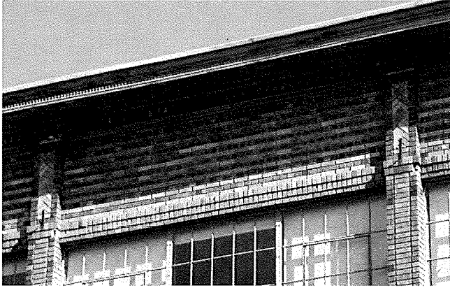
Figure 2. South Elevation; note dentils and decorative piers.
