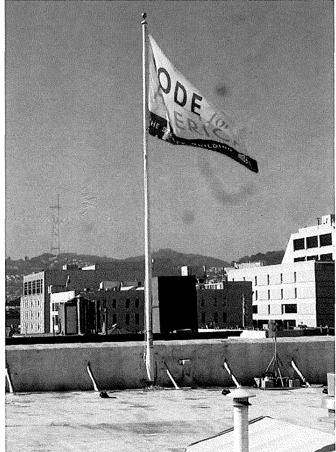
Figure 1. Flagpole along west elevation.
