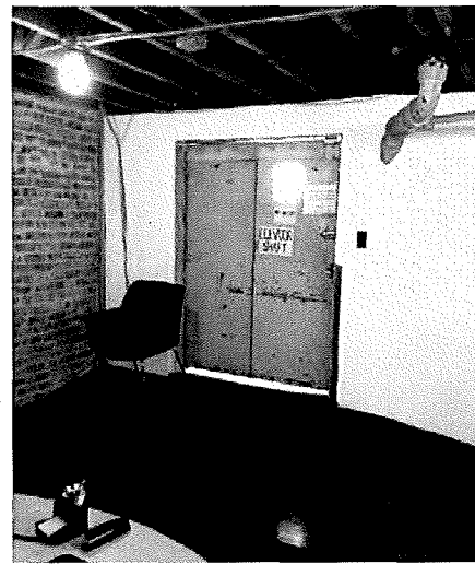
Second floor entrance to elevator shaft. (Page & Turnbull, April 2013)
