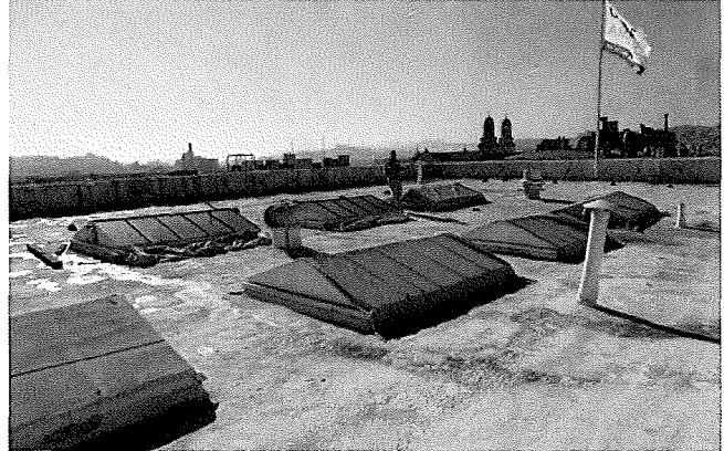
Figure 1. Roof overview; note skylights.
