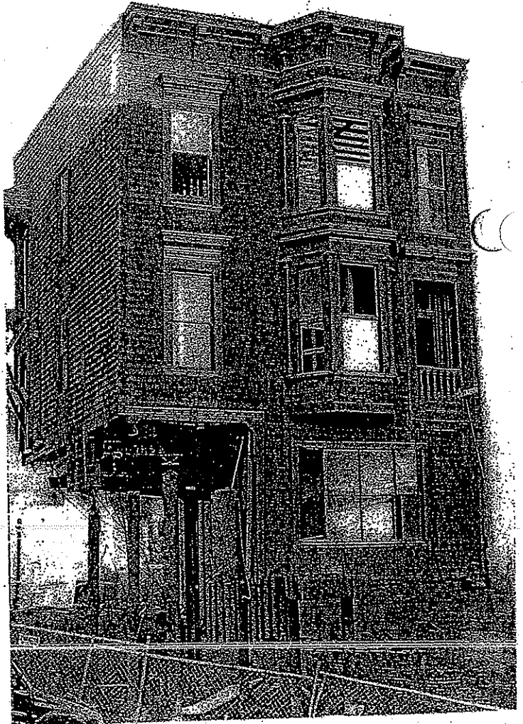
At right: The same building in early 2000, resting on steel columns and awaiting further construction.
