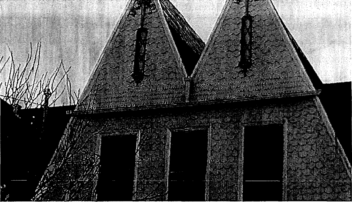
ABOVE: Detail of repaired guttering (scope 1) as well as upper vinyl windows to be replaced (scope 2)
