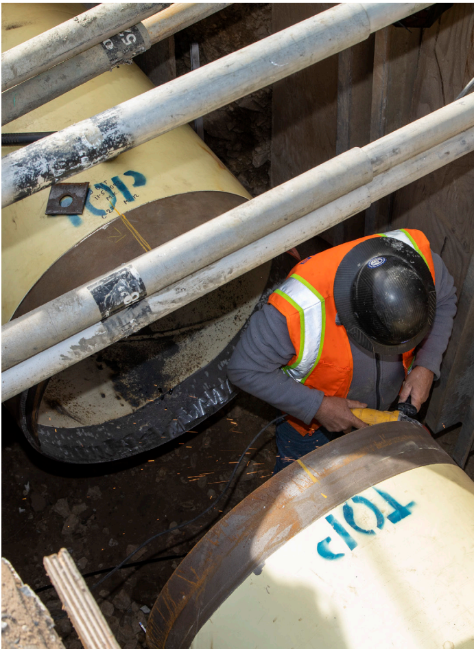
New pipeline work for Potable Emergency Firefighting Water System at 19th Avenue and Sloat Boulevard
