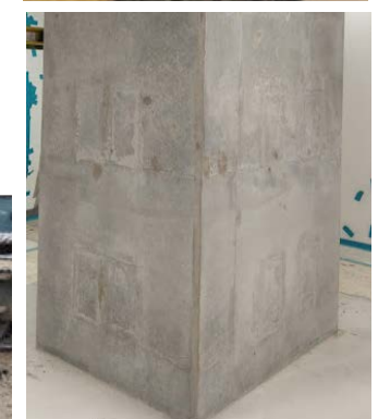
ZSFG Seismic – Column Strengthening
