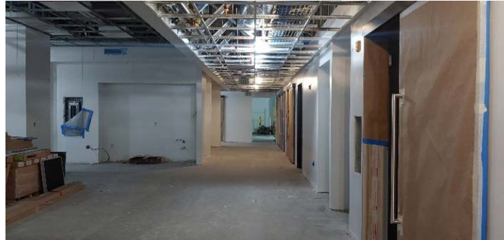
ZSFG Rehab – New Exam Rooms
