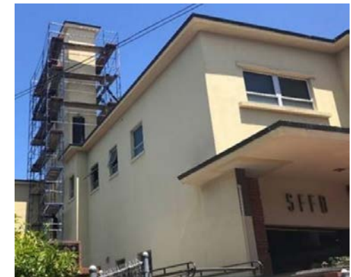
Fire Station - Seismic Hose Tower
