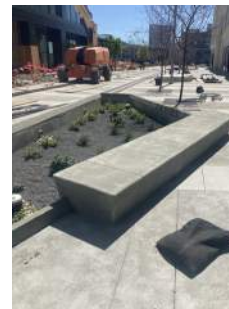
SFPUC-owned bioretention planters on Dr. Maya Angelou Way (including seatwalls integrated into the planter structure) are not subject to this IMEP.
