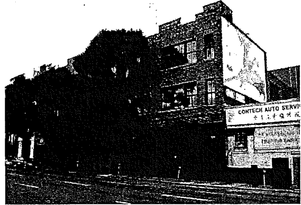
291 10th Street, E.W. Bennett and Co. Building (1909). (Page & Turnbull, October 2013)
