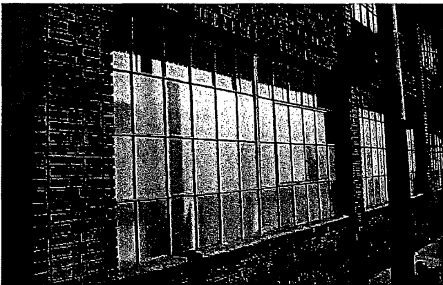
Figure 4. Typical multi-light steel windows at grade.
