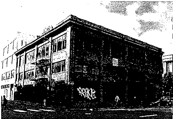
120 8 th Street, The Buzzzell Building (1925). (Page & Turnbull, October 2013)
