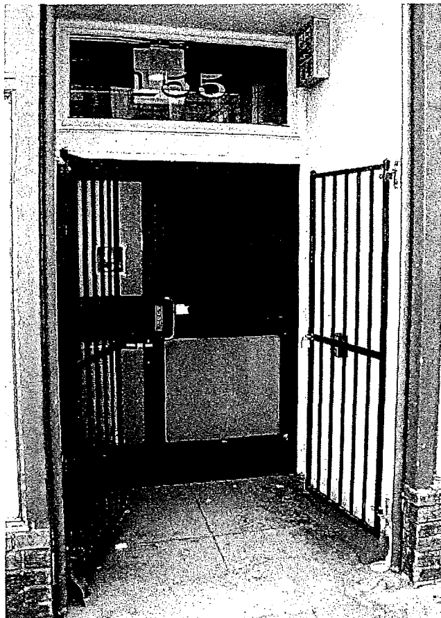
Figure 1. Metal entry door at west elevation.
