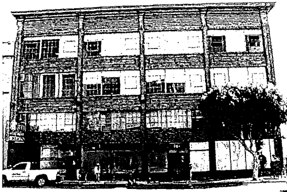
West façade facing 9 th Street. (Page & Turnbull, April 2013)
