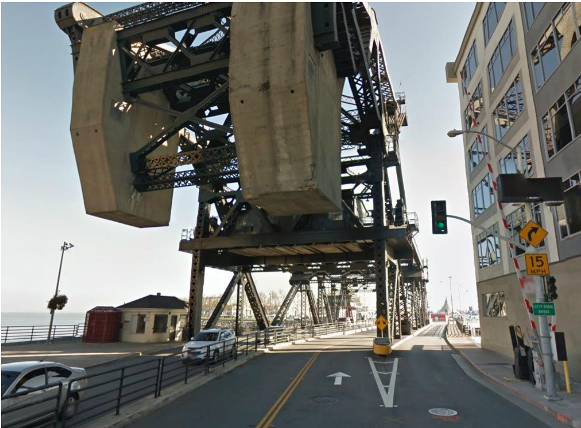
North West Corner
