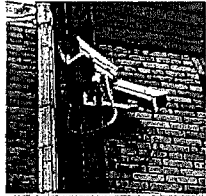
Security cameras throughout the BID
