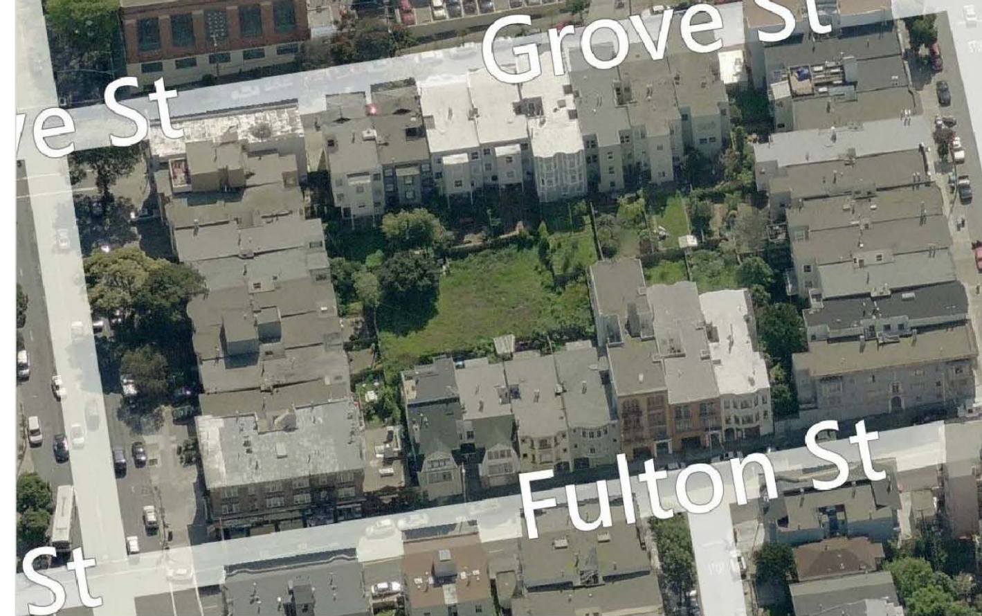
OVERHEAD VIEW LOOKING FROM SOUTH
