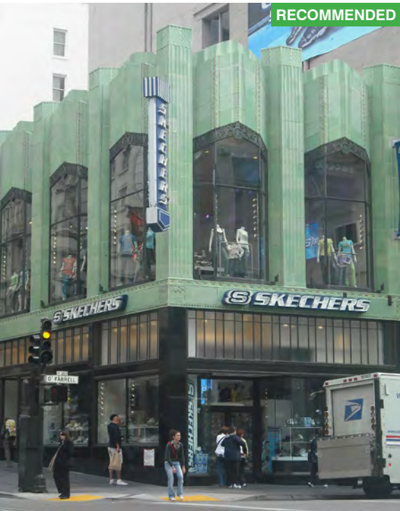
The rehabilitation project above preserved historic elements, such as the terra cotta tiles and cast iron framework. However, many other historic elements were missing, such as the transom windows and storefront pier material, were reconstructed based on historic documentation. It is common to use more than one green approach in a rehabilitation project.
